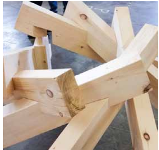
Reciprocal roof detail.
