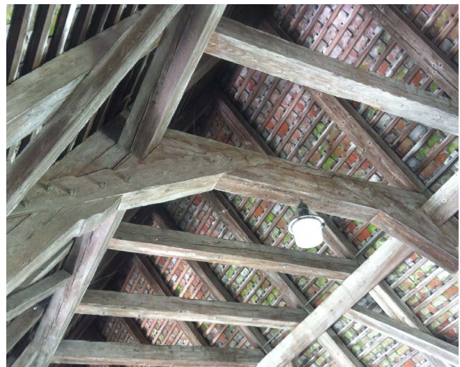
Liegender stuhl with half lapped braces.
