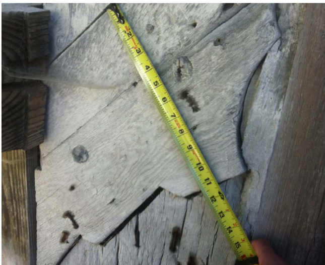
Elaborate half lap brace on a bridge.
