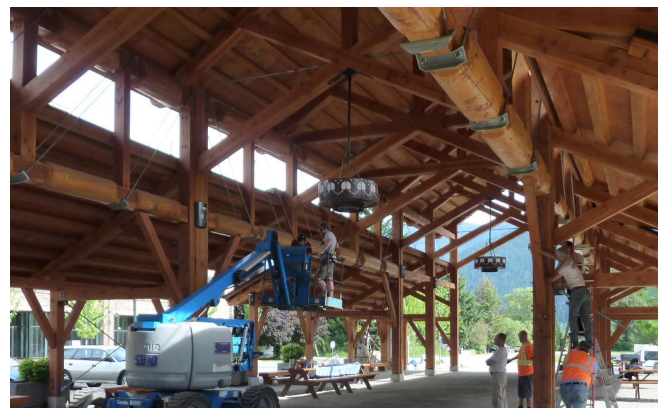
Volunteers tighten bolts and check on the barn's condition after one year.
