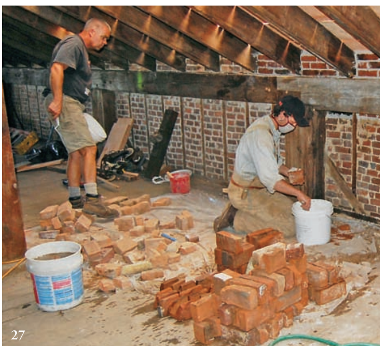
At top, left to right, Jake Amadon, Joe Miller, Joseph Ferencik and Tom Haanen coax plate into place over stud tenons. Above, Michael Murphy, left, and Will Fowlkes repair masonry infill. Below left, Tim Whitehouse checking actual needed brace length. Below right, lower end of replacement brace swung into position via overcut mortise and small chiseled relief, then blocked in tightly.
