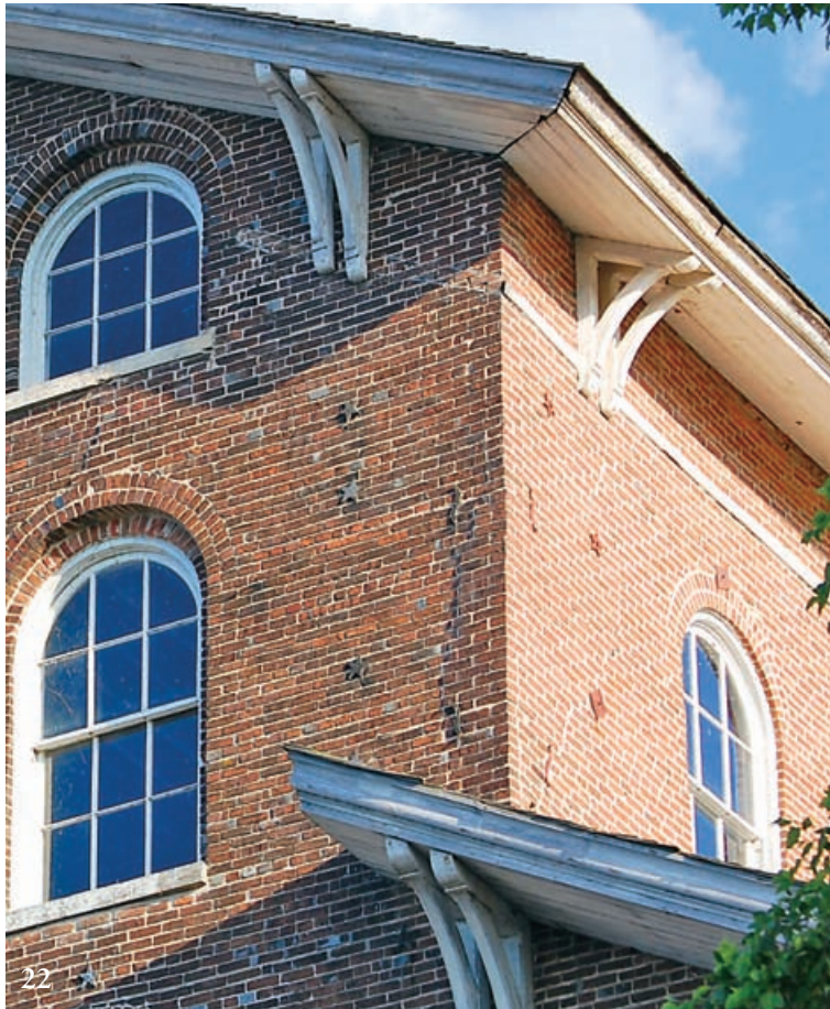
Above, cracking and distortion at monitor northwest corner, a fault in large brick buildings without expansion joints. Note star brick ties. Facing page, top left, east monitor wall, north end, with large diagonal fractures, previous repairs and distortion of brick coursing lines. Top right, west monitor wall showing rotation and misalignment of stone sills, bowing of wall below windows. Middle left, cast-iron star brick tie that held cladding to wood sheathing, across an air space. Middle right, clinching-head spike used as supplemental tie for the 4-in. brick cladding. Below left, section at top of main wall.
