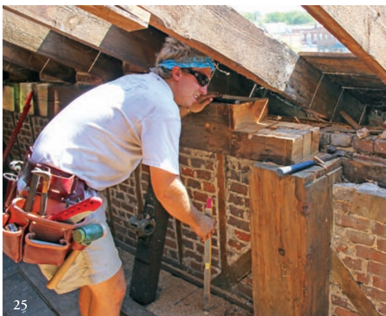
At top, section through monitor wall showing stone window sills in original position. Above, damaged brickwork resulting from tightening 1 1/4-in. iron rods against an air space. Below, Jared Wilson prepares for scarfed-in plate repair.
