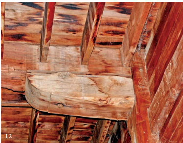
At top, typical interior post with oak bolster. Notch in bolster may reflect clearance for object no longer present. Note reductions on joists, stopped chamfers on beam and post as well as stepped profile of bolster, all signs of conscious craftsmanship. Above, tenoned half-bolster at exterior post, through-bolted to girder. Below, plan and elevation views of bolstered girder joint at post.
