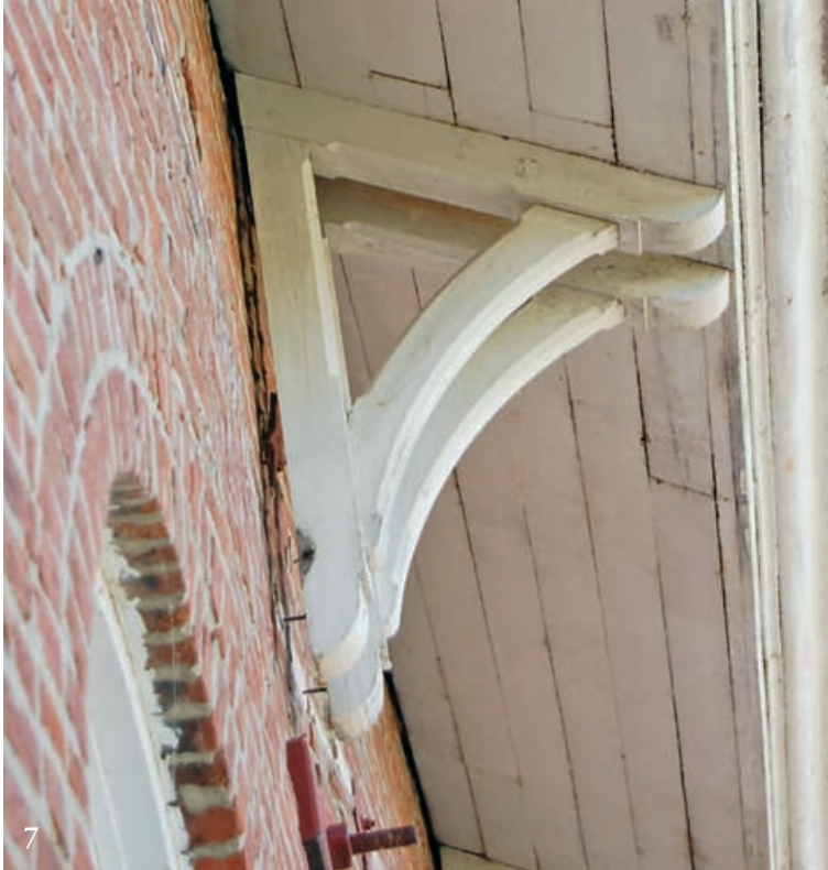
Above, decorative bracket separated from wall. Below, multistory grain bins, independently supported down to foundation.
