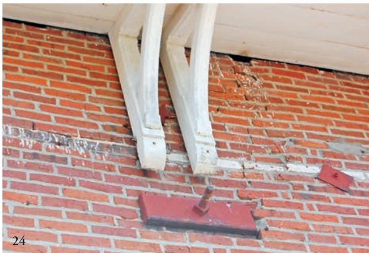
At top, section through monitor wall showing stone window sills in original position. Above, damaged brickwork resulting from tightening 1 1/4-in. iron rods against an air space. Below, Jared Wilson prepares for scarfed-in plate repair.
