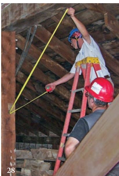
At top, left to right, Jake Amadon, Joe Miller, Joseph Ferencik and Tom Haanen coax plate into place over stud tenons. Above, Michael Murphy, left, and Will Fowlkes repair masonry infill. Below left, Tim Whitehouse checking actual needed brace length. Below right, lower end of replacement brace swung into position via overcut mortise and small chiseled relief, then blocked in tightly.
