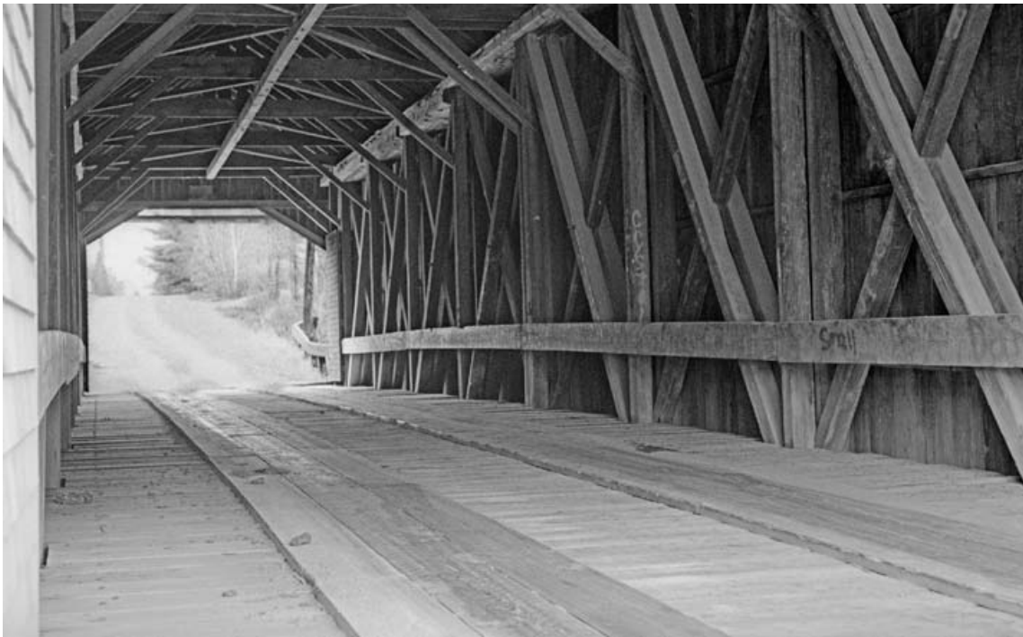
Fig. 9 Robyville bridge, Corinth, Maine (1876), span 97 ft., is very close to the Long truss patent, except that the floor has been replaced with steel beams in recent years.
