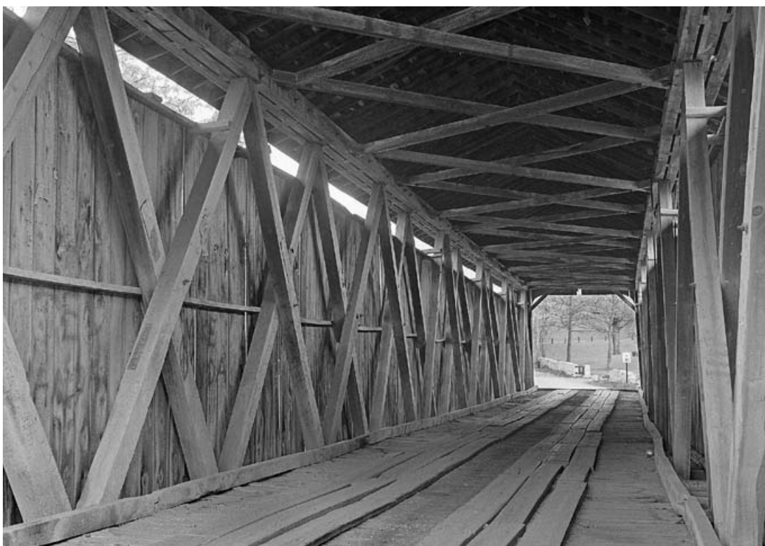
Fig. 12 Cataract Falls, Indiana, has this fine example of the Smith truss (1876), with a 150-ft. span.
