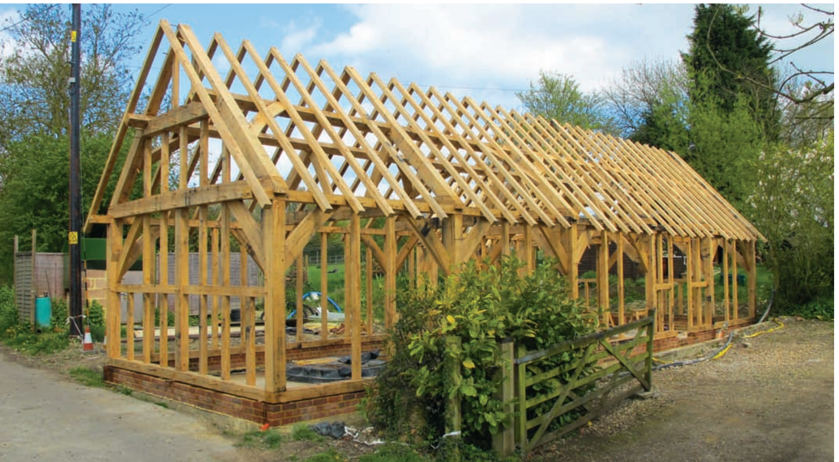
Figs. 1 and 2 At top, hoisting a principal rafter reduced to fit collar seen just behind and to clasp a purlin yet to be offered. Above, three-quarter view of a frame that might have existed in Hertfordshire in the 17th century. Clasped purlins can be seen at gable end.
