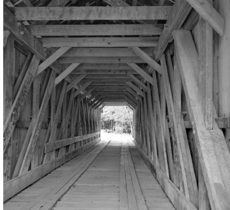
Fig. 16 Bunker Hill bridge (1895), 81-ft. span, Catawba County, North Carolina, the last Haupt truss in existence.
