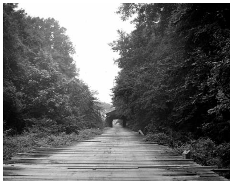
Fig. 7 The floodplains of southern rivers and creeks often required long raised approaches to meet the bridge, here Red Oak Creek bridge (ca. 1840, 127 ft.) in Meriwether County, Georgia.
