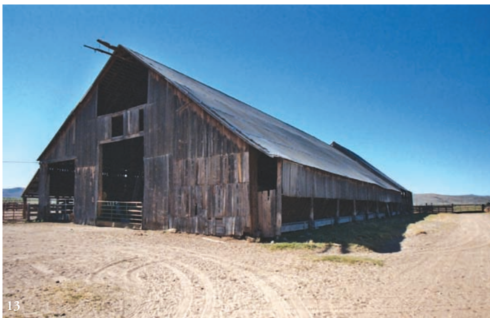
Fig. 10 At top left, Gansberg barn, Woodsford, California, ca. 1910. Partial view of central aisle and one side aisle. Hewn Ponderosa pine. Note cut sill (for tractor passage) and empty brace mortise.
