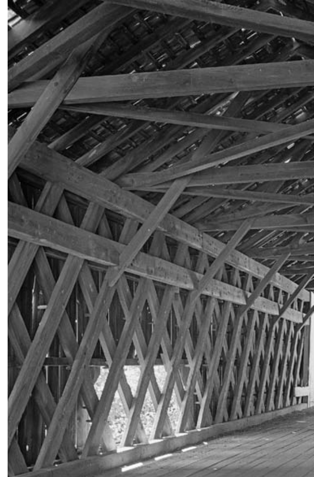
Fig. 6 Bridge over the Delaware Canal at Uhlerstown, span 110 ft. Most regions of Pennsylvania used the Burr
