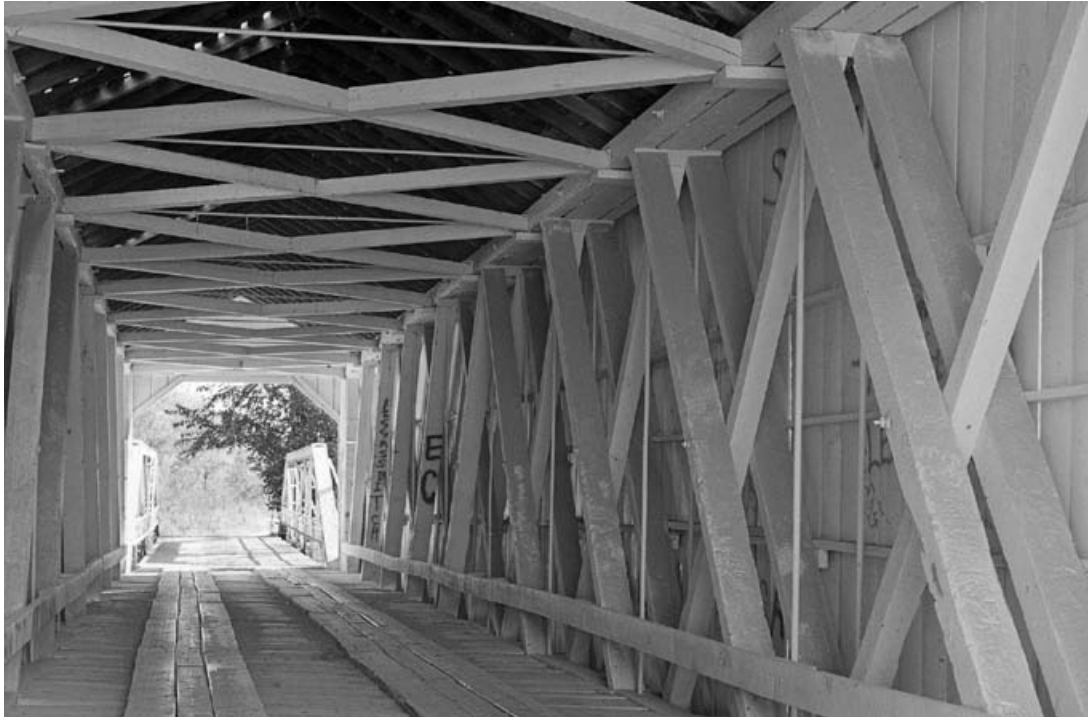
Fig. 11 The former Wolf bridge over the Spoon River in Knox County, Illinois (1874), span 106 ft., was a classic example of the Howe truss.
