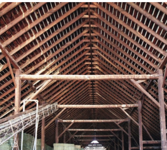
Fig. 10 At top left, Gansberg barn, Woodsford, California, ca. 1910. Partial view of central aisle and one side aisle. Hewn Ponderosa pine. Note cut sill (for tractor passage) and empty brace mortise.
