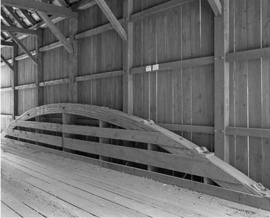
Fig. 15 Brownsville bridge, Windsor County, Vermont (date unknown), 45-ft. span, supported by a simple tied arch.
