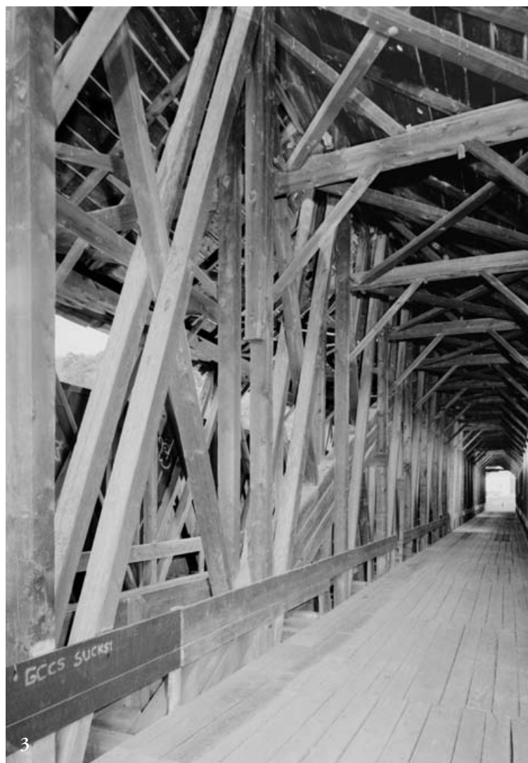
Fig. 2 View of uppermost part of central truss, with clasped arch running just below ridge of bridge roof and showing wedged connections for lateral and transverse braces and truss counterbraces.
