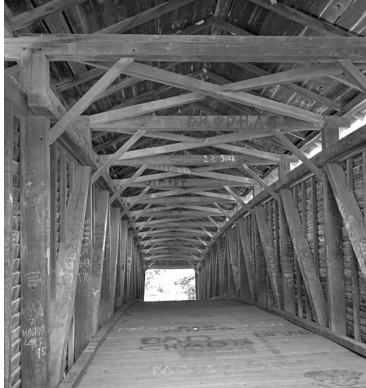
Figs. 13, 14 Humpback bridge near Covington, Virginia (1857), span 106 ft., uses a multiple kingpost truss with arched chords.
