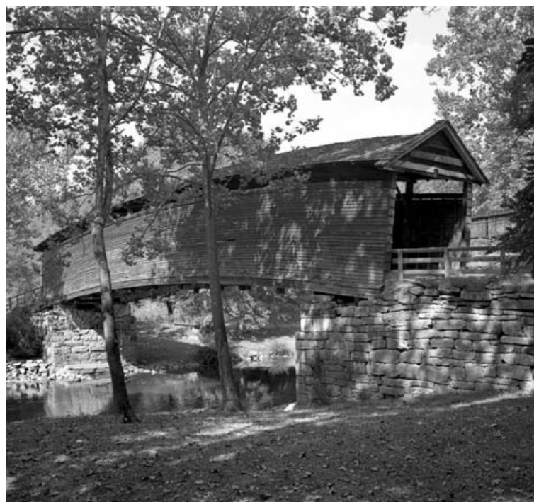
Figs. 13, 14 Humpback bridge near Covington, Virginia (1857), span 106 ft., uses a multiple kingpost truss with arched chords.
