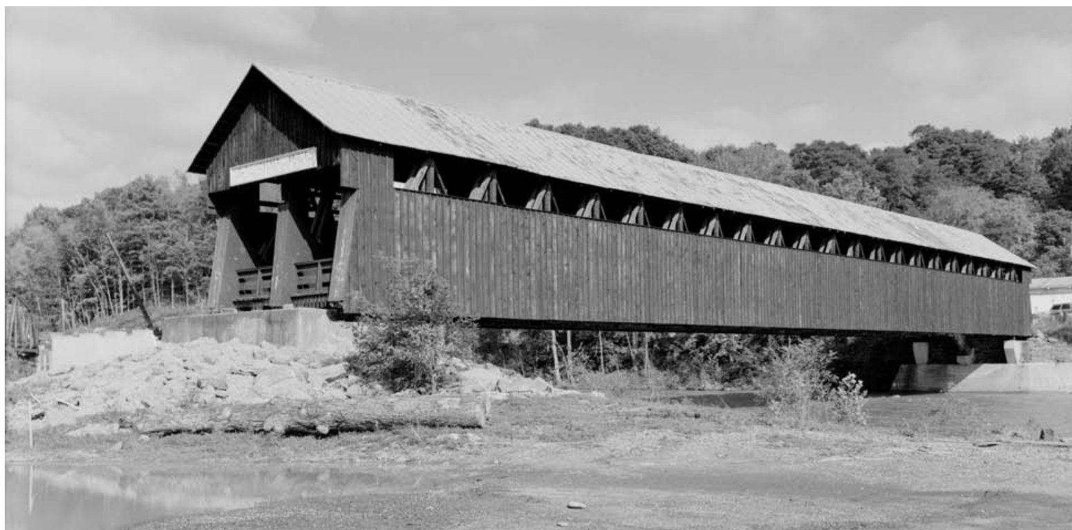
Fig. 1 The Blenheim bridge over the Schoharie Creek, North Blenheim, New York, 210-ft. clearspan, built 1855, destroyed 2011. It served road traffic until the 1930s, when it was supplanted by a steel bridge.
