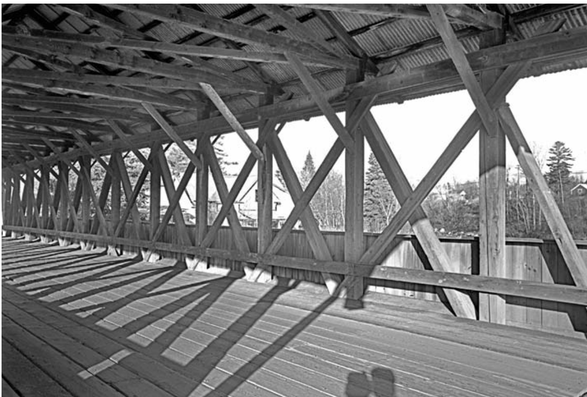
Fig. 10 Mechanic Street bridge over the Israel River in Lancaster, New Hampshire (1862), with a 94-ft. span, a typical Paddleford truss.
