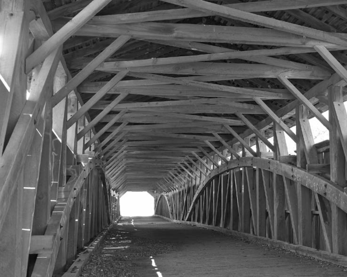
Fig. 5 Pomeroy bridge in Juniata County, Pennsylvania (1902), is a two-span Burr truss and at 278 ft. the longest covered bridge in the state.
