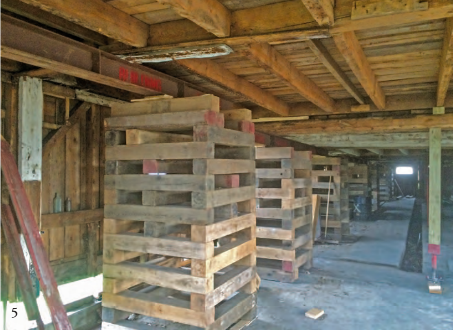
5 Lifting eaves side of barn from beneath transverse sills with steel brackets to bring load to outside wall. Notice pyramid arrangement of cribbing at top of tower in foreground.
