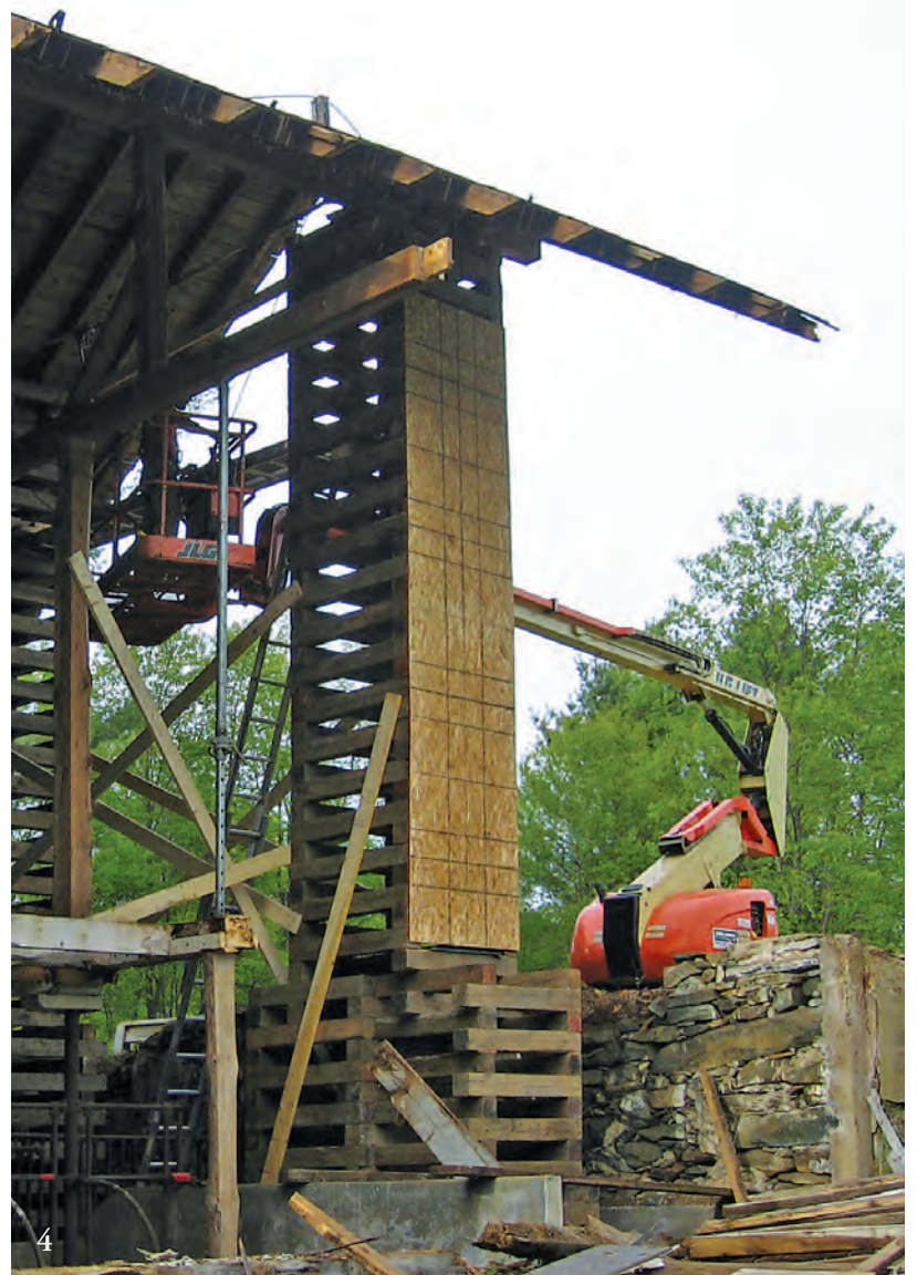
3 Paired, braced 26-ft. towers sheathed on two faces support failing gable end of barn at purlins, first 7 ft. built twice as long for stability. Slates first removed from lower half of roof.
