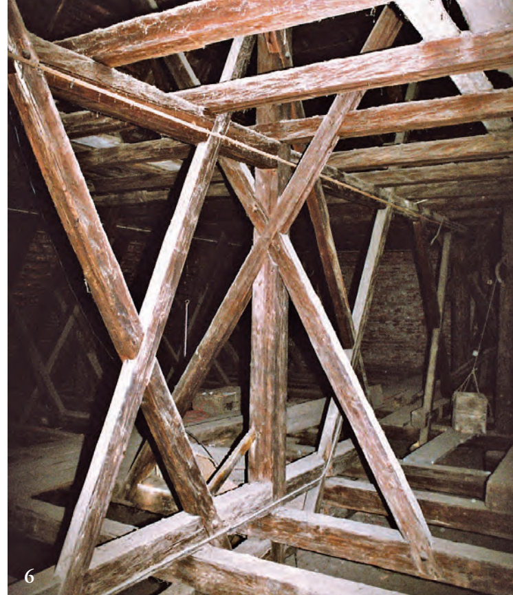
5 St. Andrew in Leoben-Göss, junction of second lowest collar beam with post and crossed braces in frame type A. Lap joints allow assembly only in a certain sequence.
