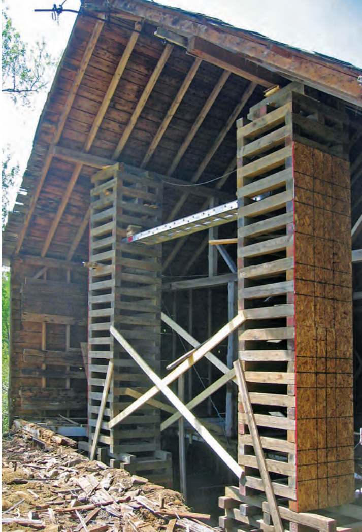
3 Paired, braced 26-ft. towers sheathed on two faces support failing gable end of barn at purlins, first 7 ft. built twice as long for stability. Slates first removed from lower half of roof.
