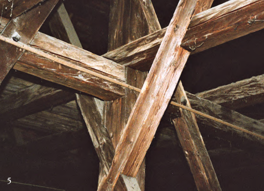
5 St. Andrew in Leoben-Göss, junction of second lowest collar beam with post and crossed braces in frame type A. Lap joints allow assembly only in a certain sequence.
