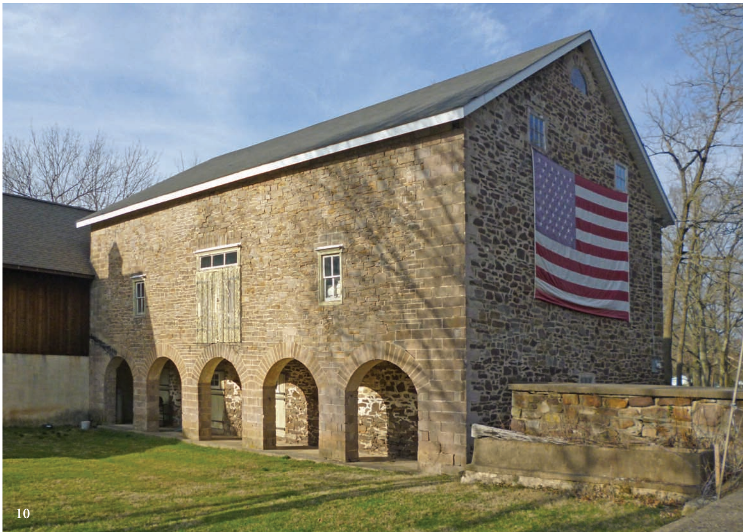
10 Stone-arch forebay barn 38 ft. x 53 ft., near Edison, Bucks County, Pa., ca. 1830. Built for Dr. Samuel Moore, who was Quaker, and remarkable for its rare dressed stone work. Stone arch form is likely of English origin.
