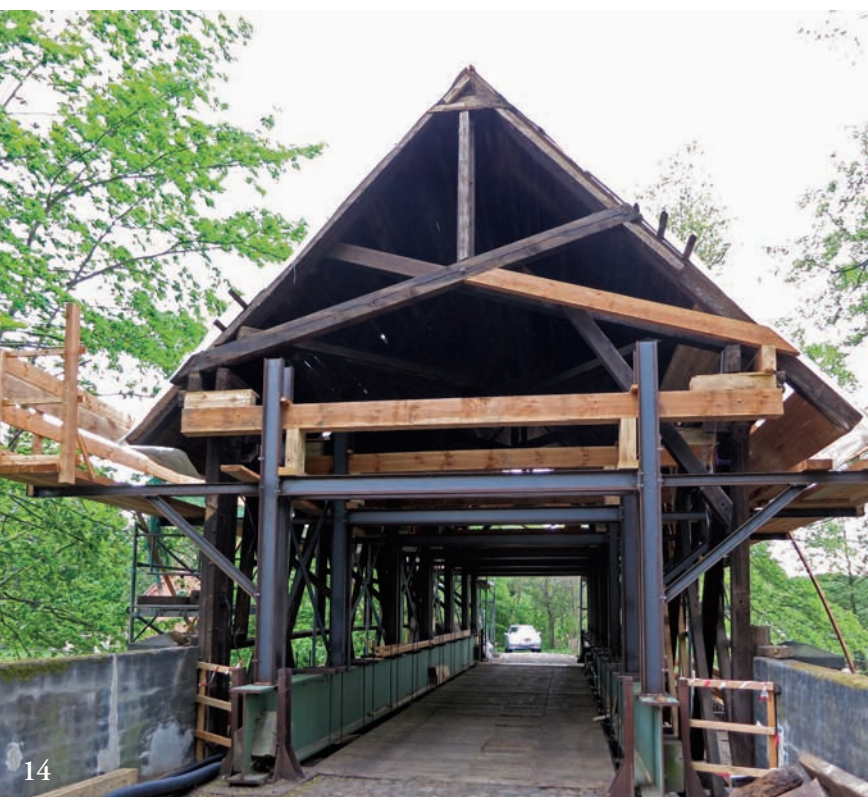
12 Lower gantry outside trusses with simple boarded walkways on long baulks of timber resting on lower chords. Until trusses were completed, lower chords were suspended from floor beams.
