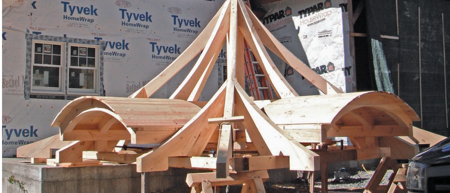
1 Cupola under construction for house in central Vermont.
