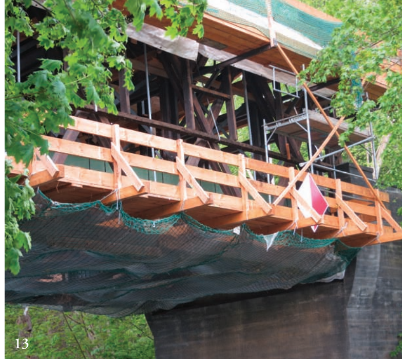
12 Lower gantry outside trusses with simple boarded walkways on long baulks of timber resting on lower chords. Until trusses were completed, lower chords were suspended from floor beams.
