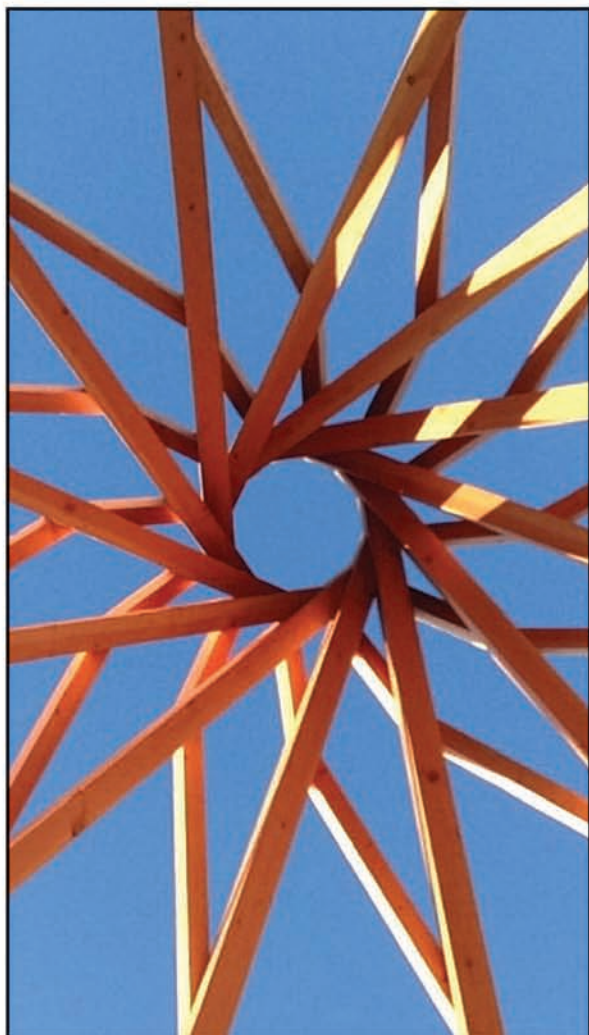
Reciprocal roof framing at the St. James Episcopal Church in Cannonball, ND by Empire Timberworks.
