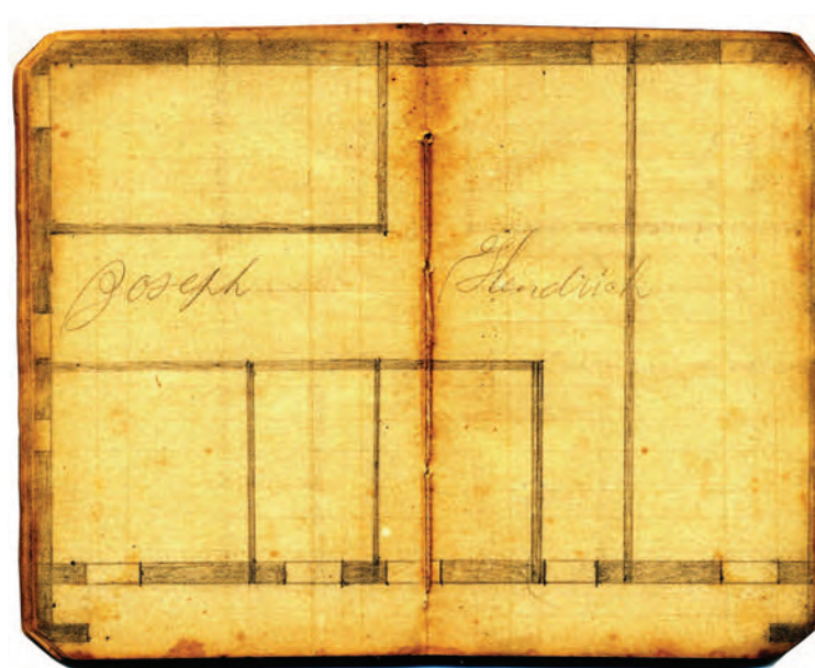
6 Basement plan for Henrich (here Hendrich), showing stable layout with feed aisle and Peilereck closures at forebay ends.
