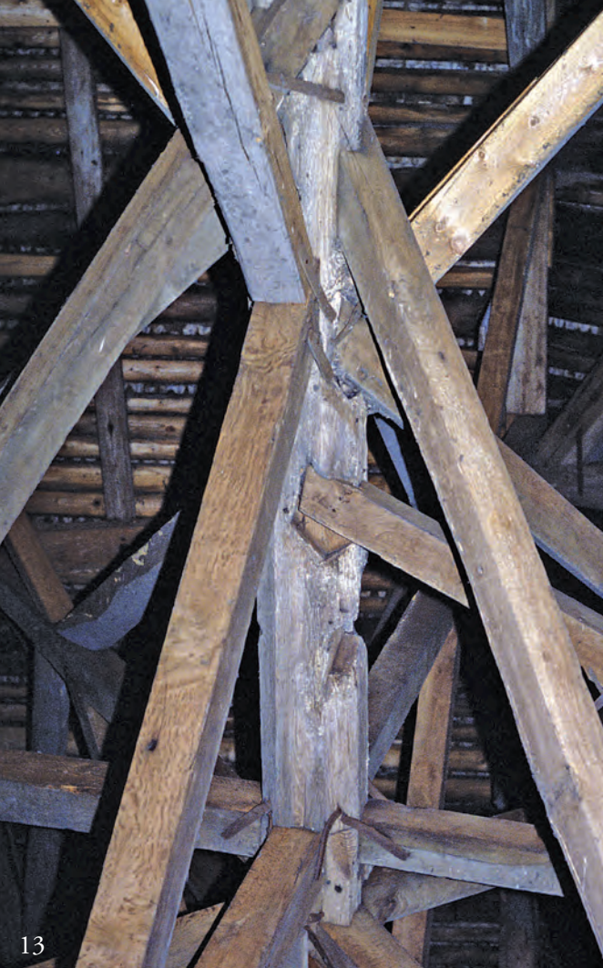
13 Replacement 19th-century collars join mast awkwardly in upper half of second stage.
