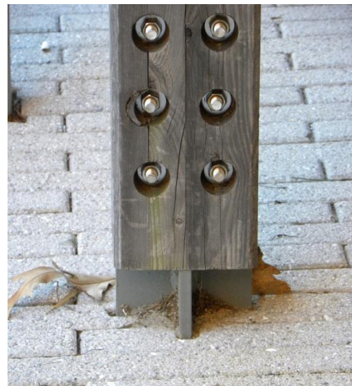
Figure 11 Elevated post base drains freely
