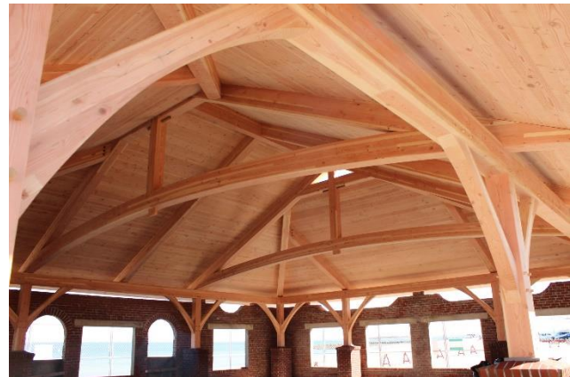
Figure 1 A glulam timber structure with traditional joinery and a CLT roof deck
