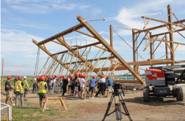
Harris Barn Restoration, 2012, Delta, B.C.
