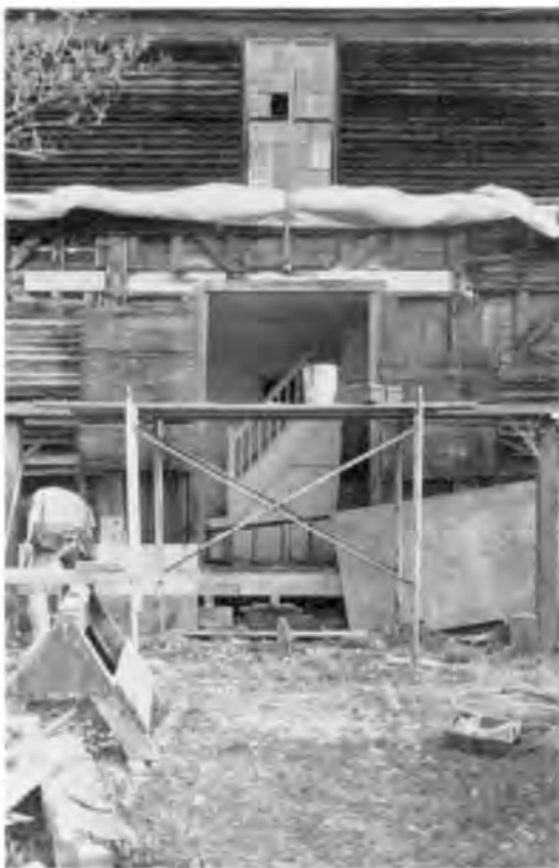
Above and below, work at the Theron Boyd house, built 1787 at Quechee, Vermont, and now owned by the state, called for preservation undisturbed of the original interior. Most repairs were thus carried out from the exterior. Shown here are new beech sills joined to the old and a glimpse of the interior. The jacking plate in the photo above is bolted to every post and stud.
