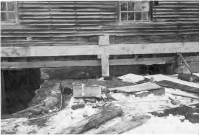
Above and below, work at the Theron Boyd house, built 1787 at Quechee, Vermont, and now owned by the state, called for preservation undisturbed of the original interior. Most repairs were thus carried out from the exterior. Shown here are new beech sills joined to the old and a glimpse of the interior. The jacking plate in the photo above is bolted to every post and stud.
