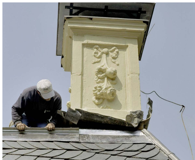
Flashing on Dutch chimney restoration.
