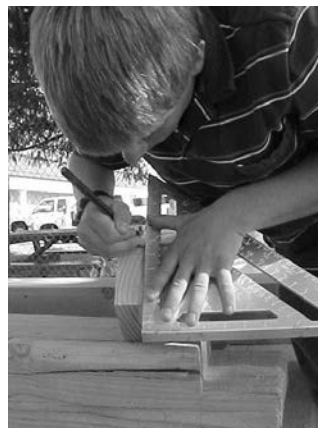
Spencer Oldemeyer laying out a tenon.
