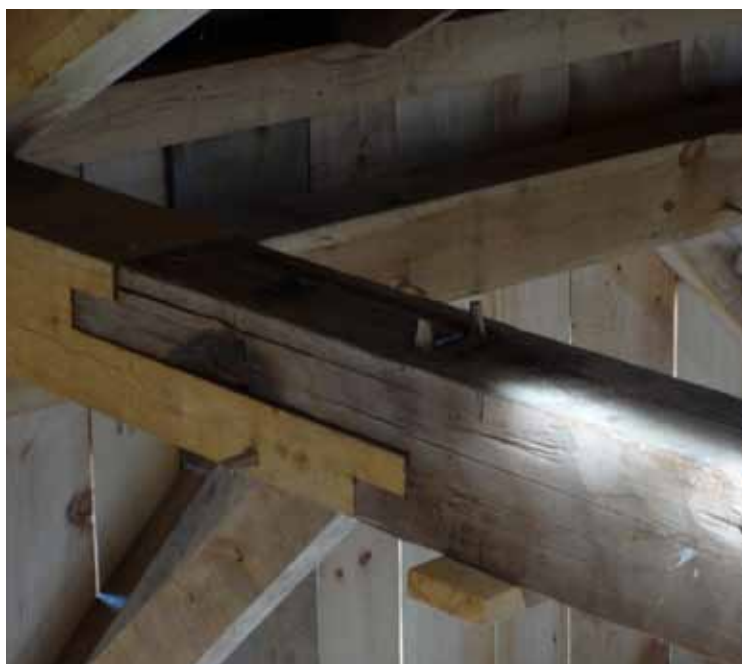
Sanborne's main barn, which experienced a fire and is in restoration. Bladed scarf joint is clamped by central bolt unseen in deep shadow.
