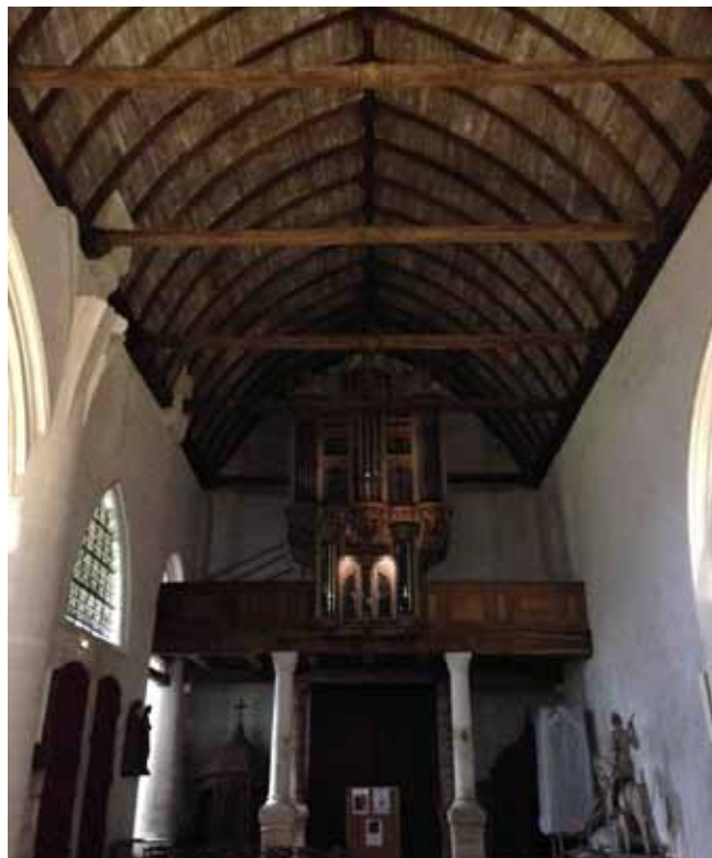
Boarded ceiling ( charpente lambrissée ) in church with pointed barrel vault.
