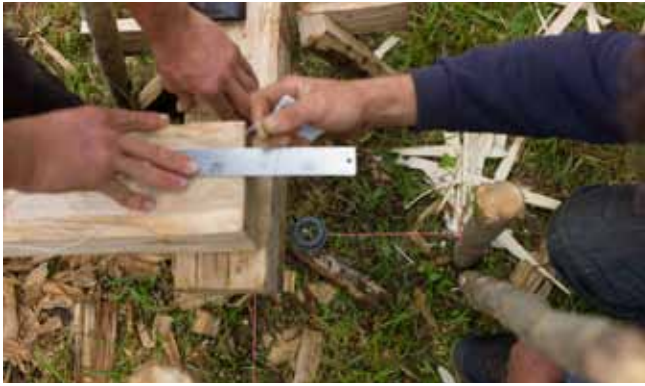
Scribing timbers with ground lines and the plumb bob.
