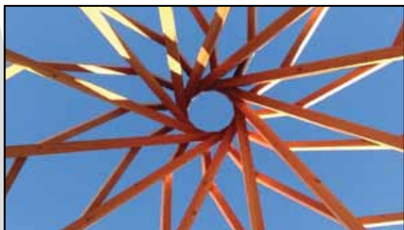
Reciprocal roof framing at the St. James Episcopal Church in Cannonball, ND by Empire Timberworks.
