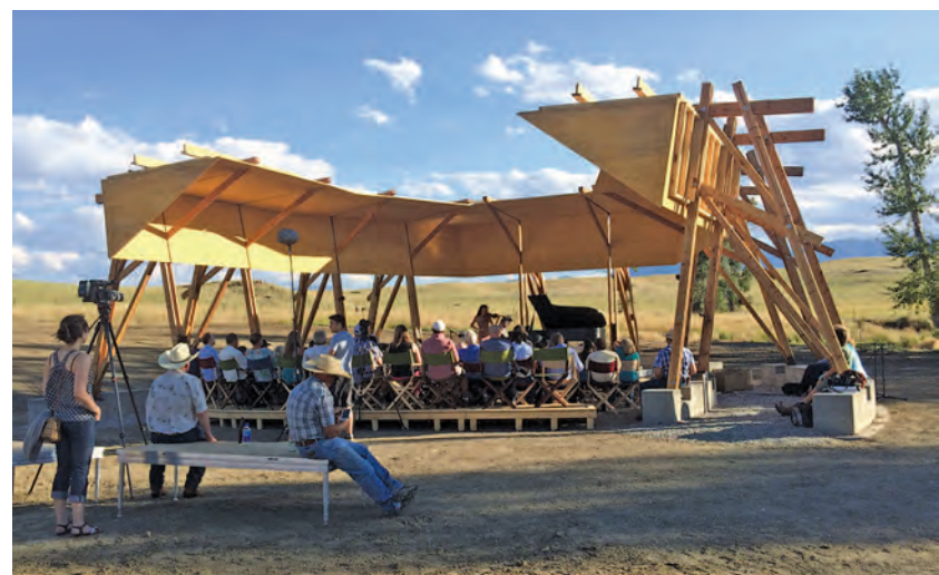
At right, acoustic shell, Tippet Rise Art Center, Fishtail, Mont., 1900 sq. ft., of Douglas fir and marine plywood. Conceptual design by ARUP, timber frame design and construction by Gunnstock Timber Frames, Powell, Wyo. Engineering by Fire Tower Engineered Timber.
