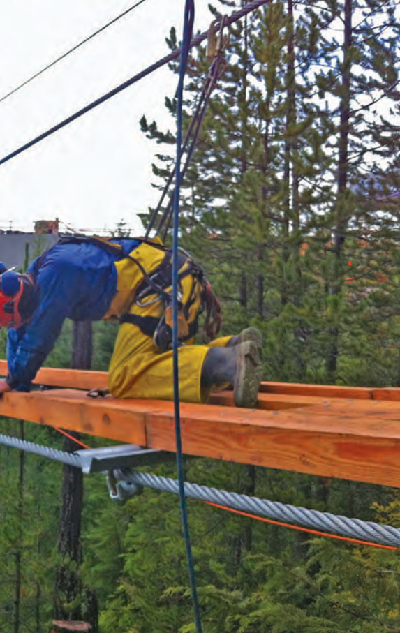
in harnesses hung directly from cables to set joists st system.
