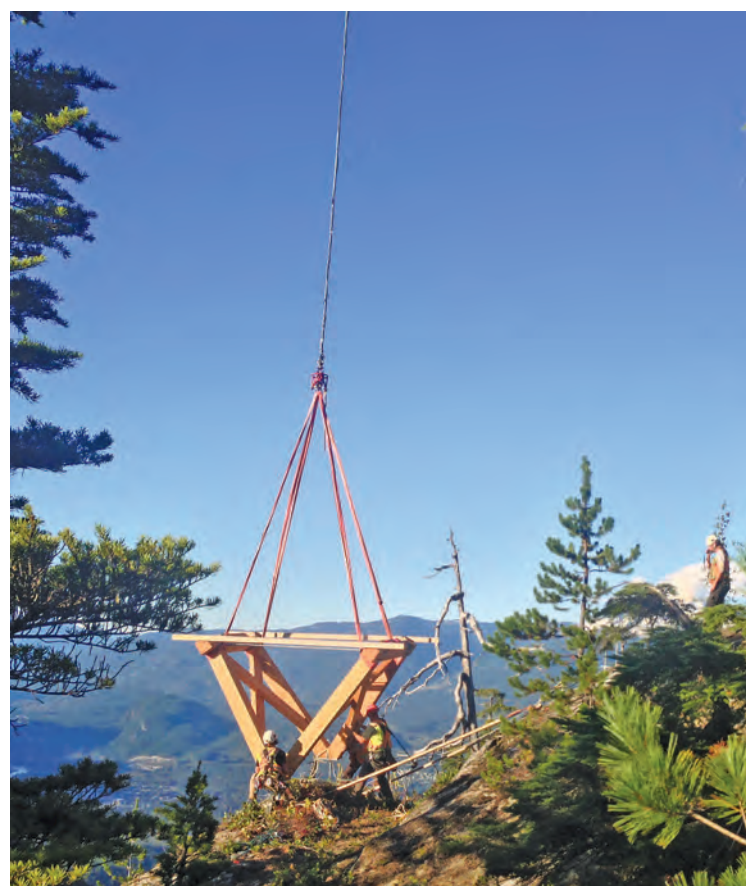
11 Setting triangular X-braced legs for Chief lookout.
