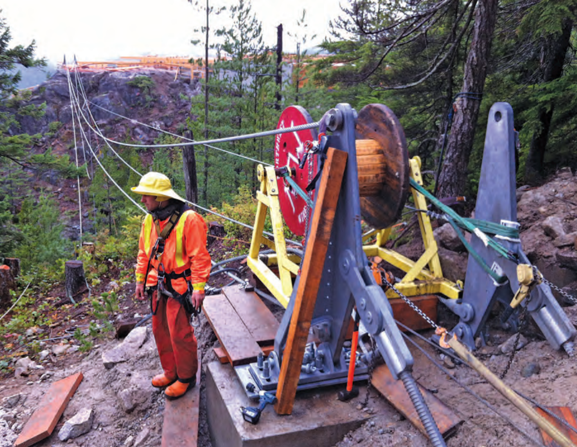
8 One of four spools of wire rope, now all paid out, successively drawn across gorge after setting initial “clothesline” with snatch block to pull cables.
