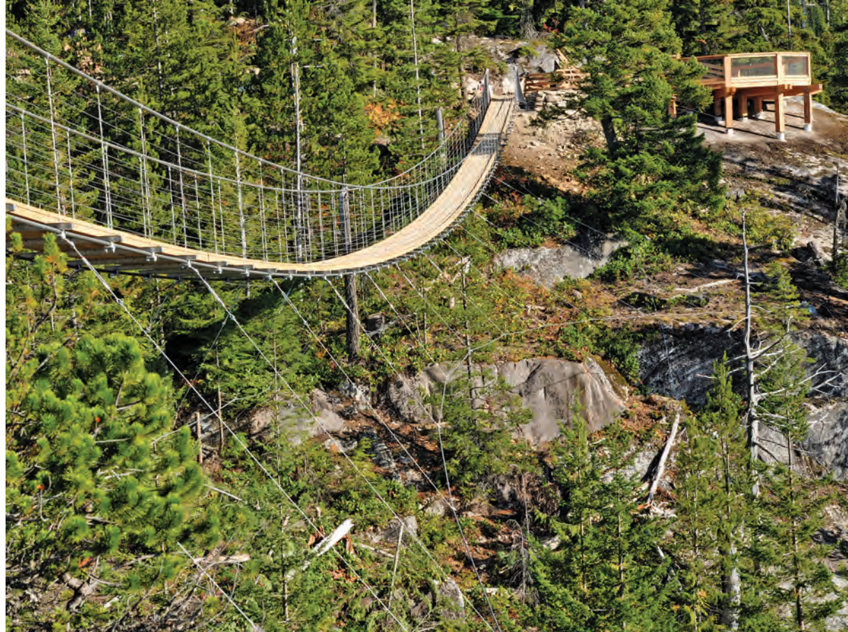
10 Completed suspension bridge is stabilized by ¼-in. guylines stretched from curving ¾-in. wire rope catenary to every third joist (15-ft. intervals).
