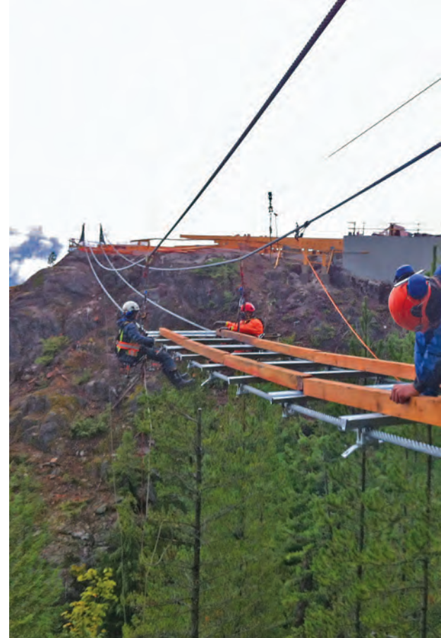
9 Installing joists and decking. Rope specialists in harness while deckers clipped into cables using fall-arrest systems.
