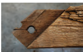
5 Brace tenon with overcut earlier shoulder line and remnant peg-hole arc.
