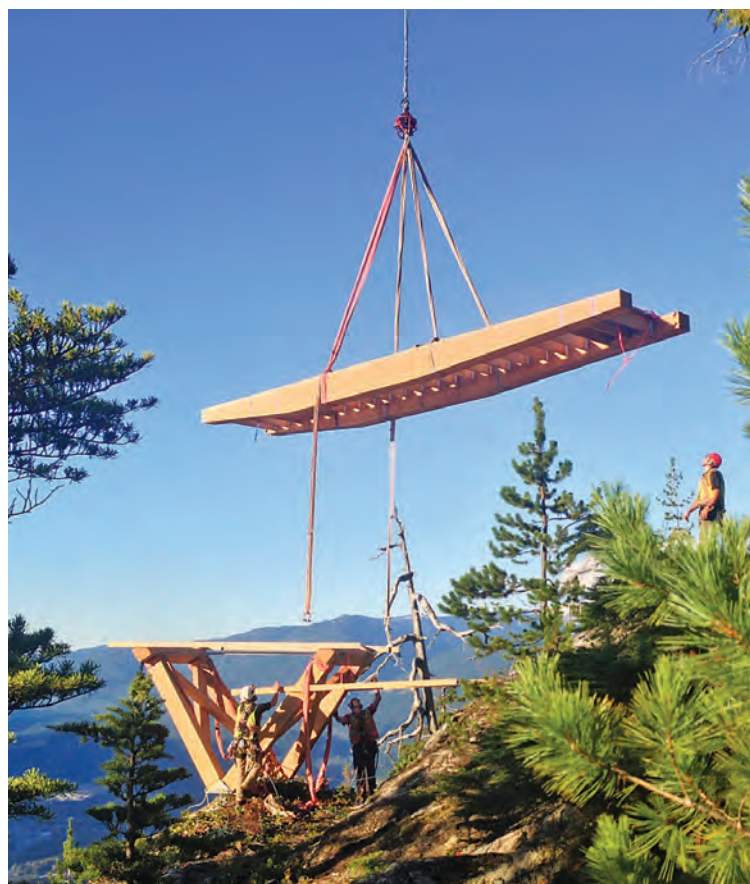
12 Heli-lifting 8 x 32-ft. deck frame for Chief lookout.
