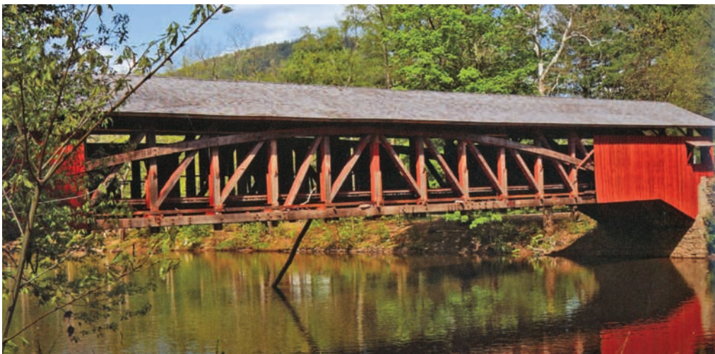
Above, 186-ft. Hillsgrove Bridge, Sullivan County, Pa., ca. 1850, typical Burr truss, siding removed for repairs.
