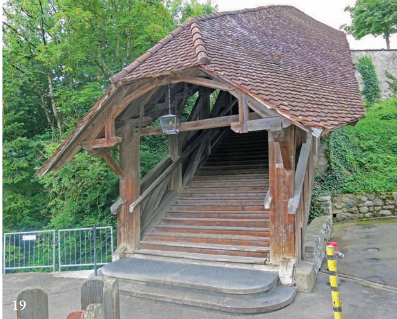
19 Erlenbach bridge portal lower end with date carved in cross beam.
