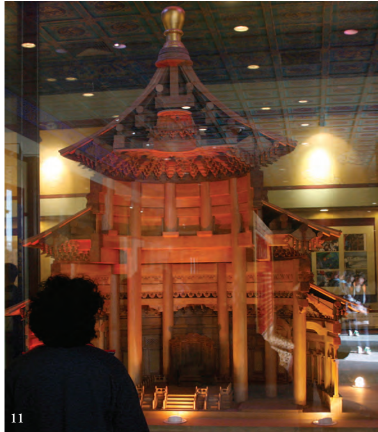
10, 11 Ch'i-nien Tien, Hall of Prayer for Good Harvest, in the Temple of Heaven, Beijing, ca. 1420, burned and rebuilt 1895, 104 ft. in diameter and 125 ft. tall. Cutaway model shows full-length coopered posts.
