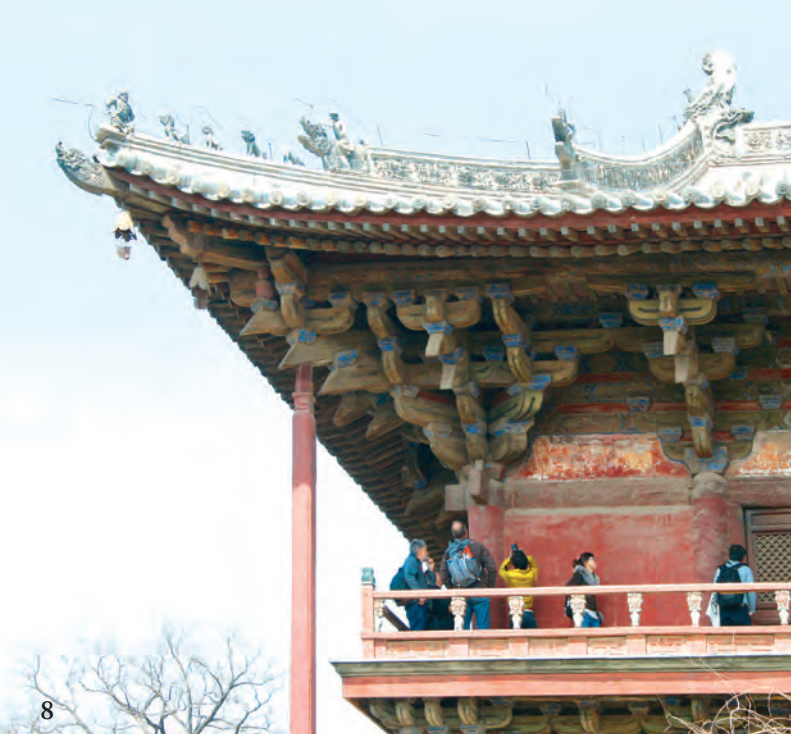
8 Massive hip brackets at Kuan-yin Ke, or Hall of Avalokiteshvara, Hopei Province, built in 984, with added post under super-extended eaves. Building has survived 32 major earthquakes.
