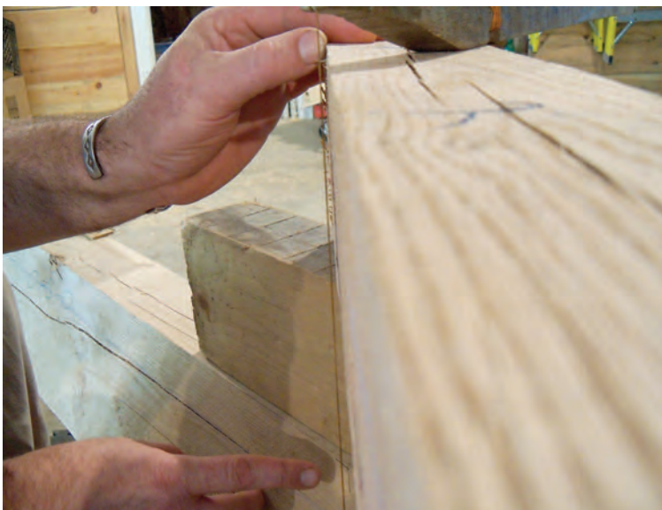
2-21 Gauging distance near A to find C.
