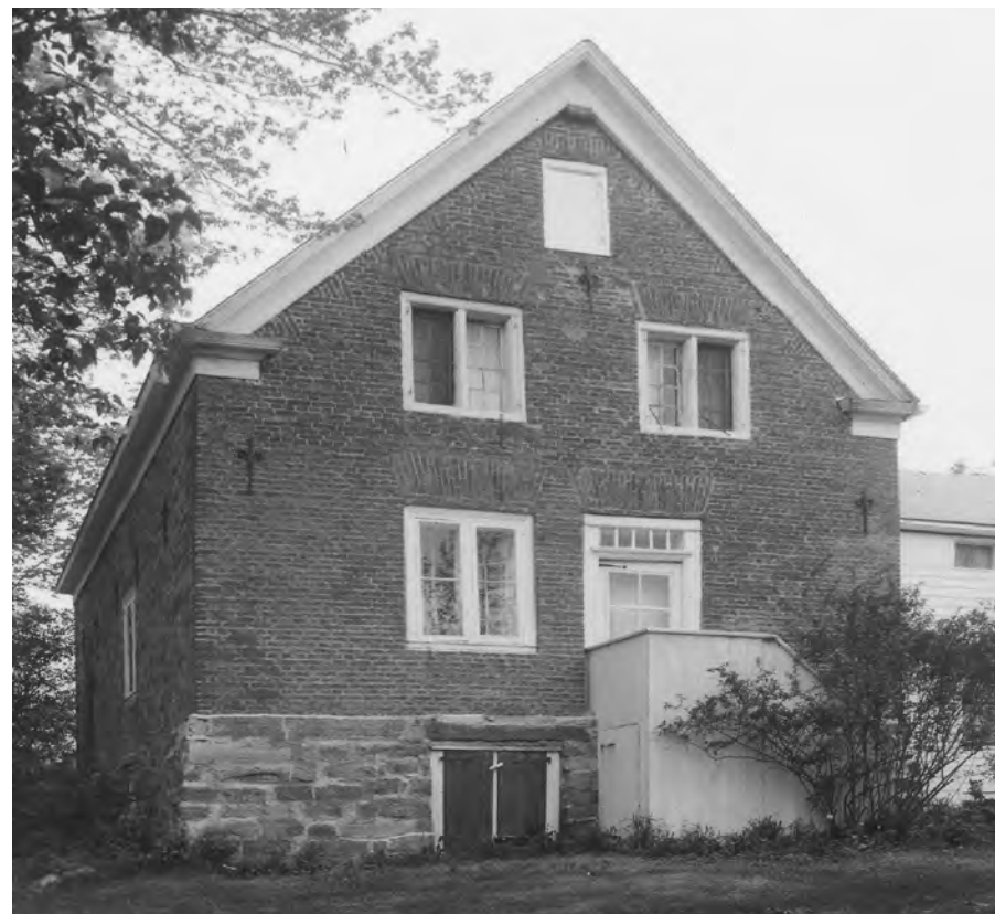
6 Teunis Slingerland house, 1762, Feura Bush, N.Y., with brick ends and stone sidewalls. Triangular brick vlechtingen follow the rake.
