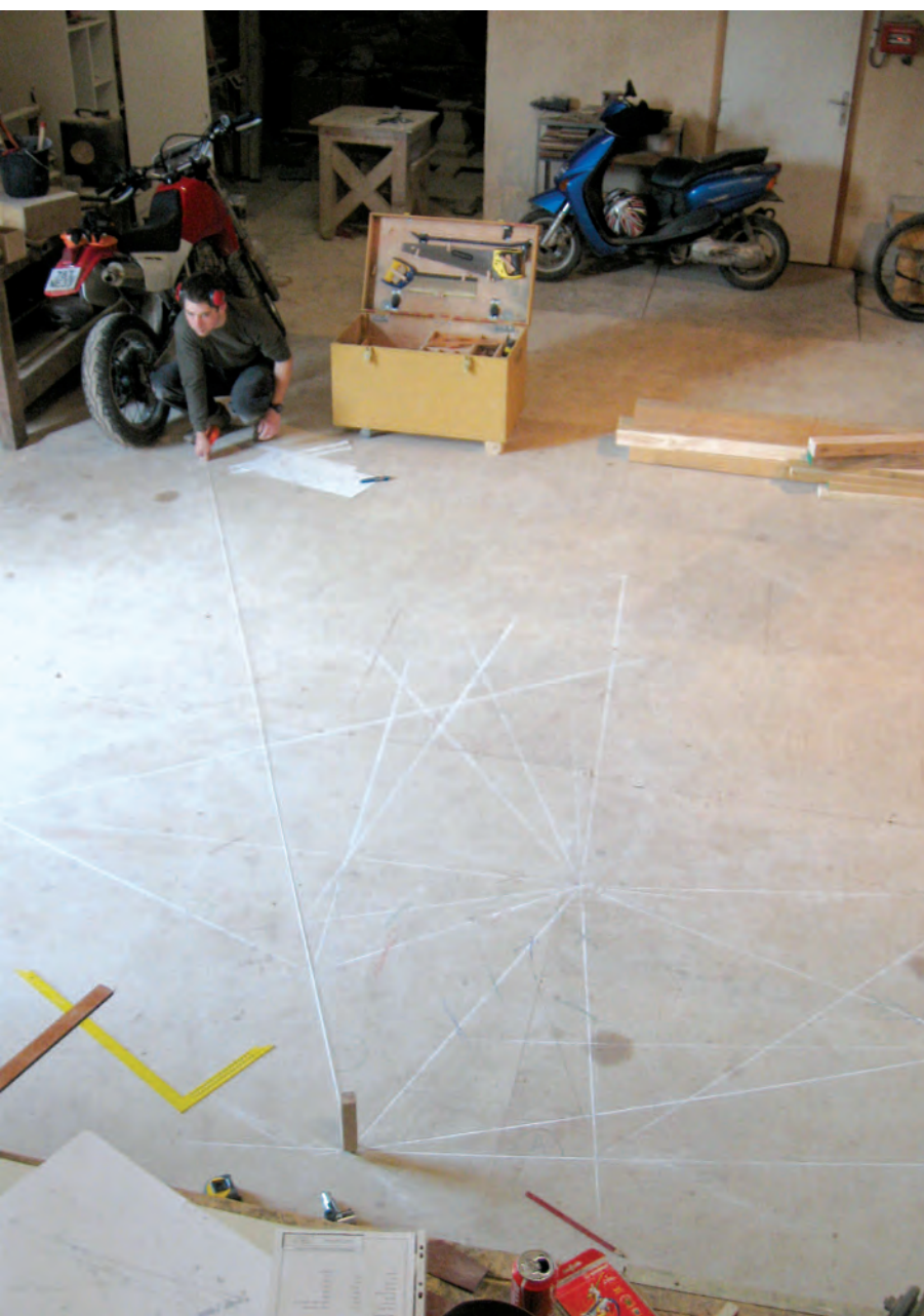
5 Aspirant carpenter "Nantais" (among motorbikes) laying out full-scale developed drawing on shop floor in Hautefort. He will build directly from drawing.
