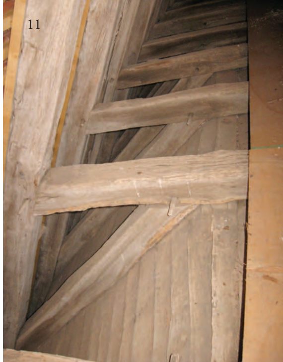
11 Detail of vault bracing to collar beams, church at Montlevicq (Indre), probably 12th century. Rafters continue down to wall plate.
