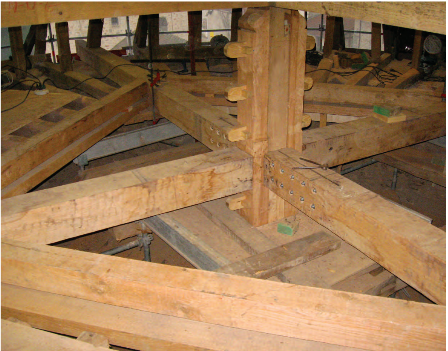
Rebuilt enrayure at 40-ft.-dia. base of oak conical roof framing in Bourganeuf (Creuse) in the Limousin region of France. Kingpost in tension hangs crossing lower chords. Fish-plates clamped to post via through-tenons and wedges provide added meat for pegging in one direction (square pegs just visible near bottom of lefthand plate); many small bolts secure spline, resisting tension in other half of crossing. Matched upper and lower horizontal struts running diagonally between chords clamp tenons of common spokes that radiate out to catch common rafter feet. Conical roofs may have several enrayures , in tension at rafter feet and in compression higher up on rafter length. Lower chords measure about 11 in. square.
