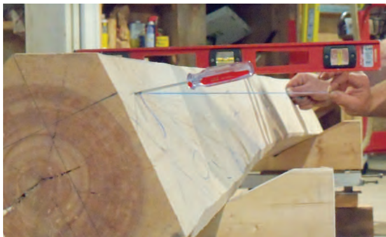
2-17 Snapping the roof offset datum line.
