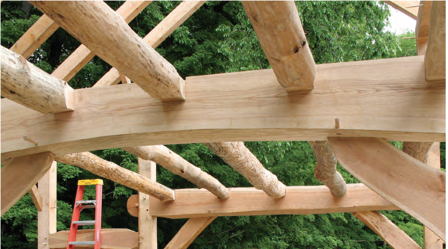
1 Student-built demonstration frame at author's building school, with white pine posts and rafters, cherry and ash tiebeams and joists of all three species, partly reflecting timber available in Berkshire Hills of Western Massachusetts.
