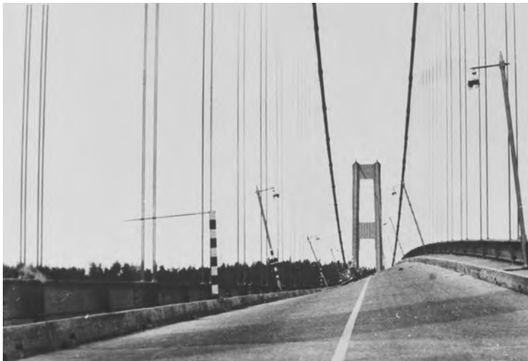
3 Tacoma Narrows Bridge, destroyed in 1940 by harmonic resonance caused by wind. Shallow deck turned out to be inappropriate design for location.
