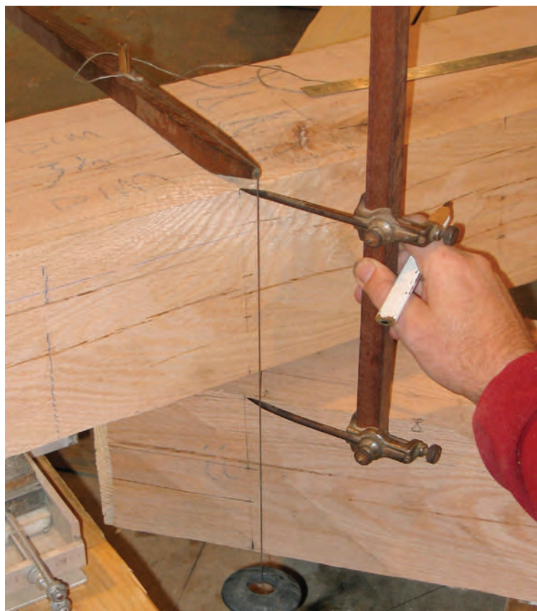
10 Using trammel points to match upper limits.
