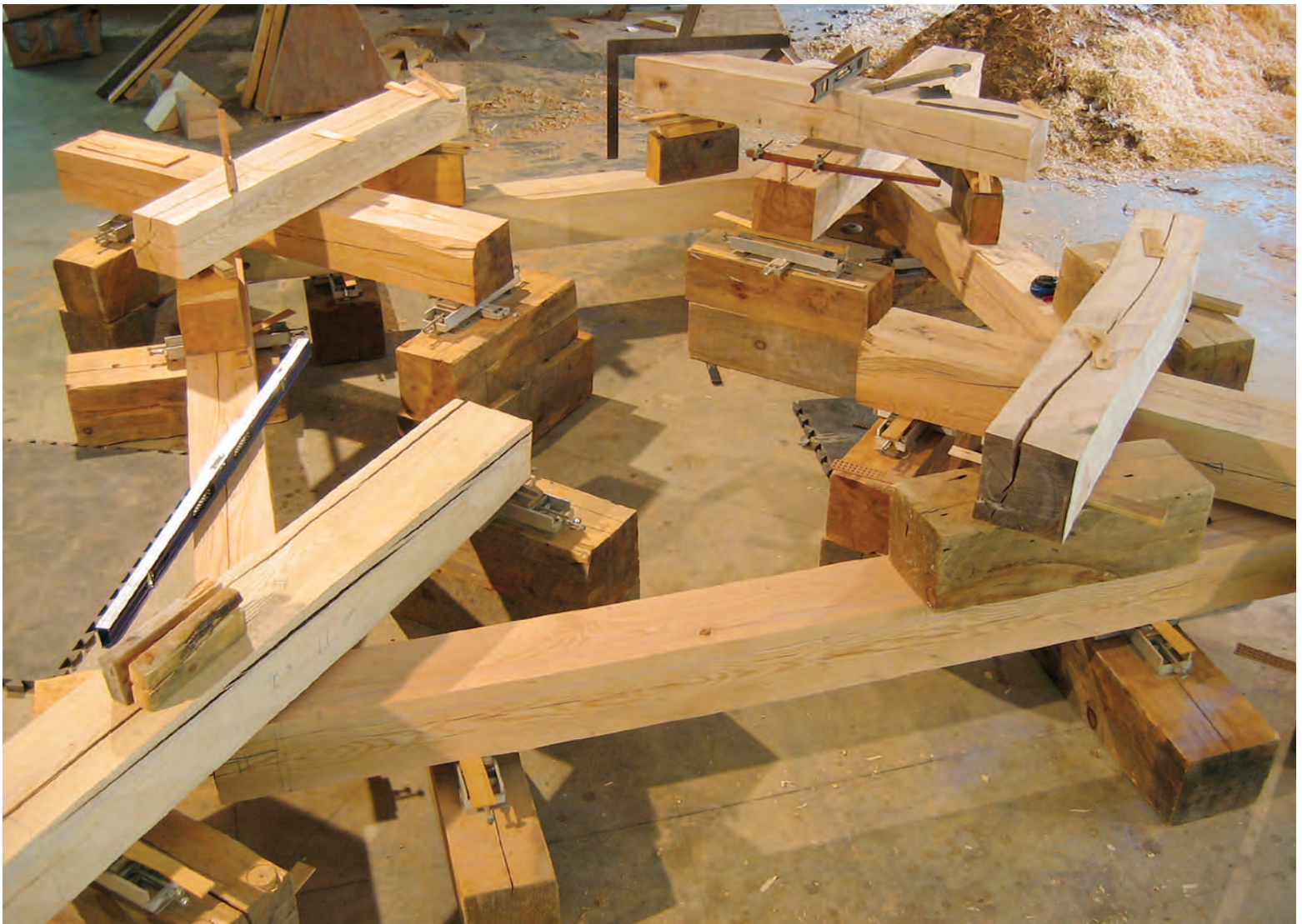
1 Layup of plate level for small structure. Scribing tool kit includes purpose-made timber-leveling devices, plumb sticks, trammel points.
