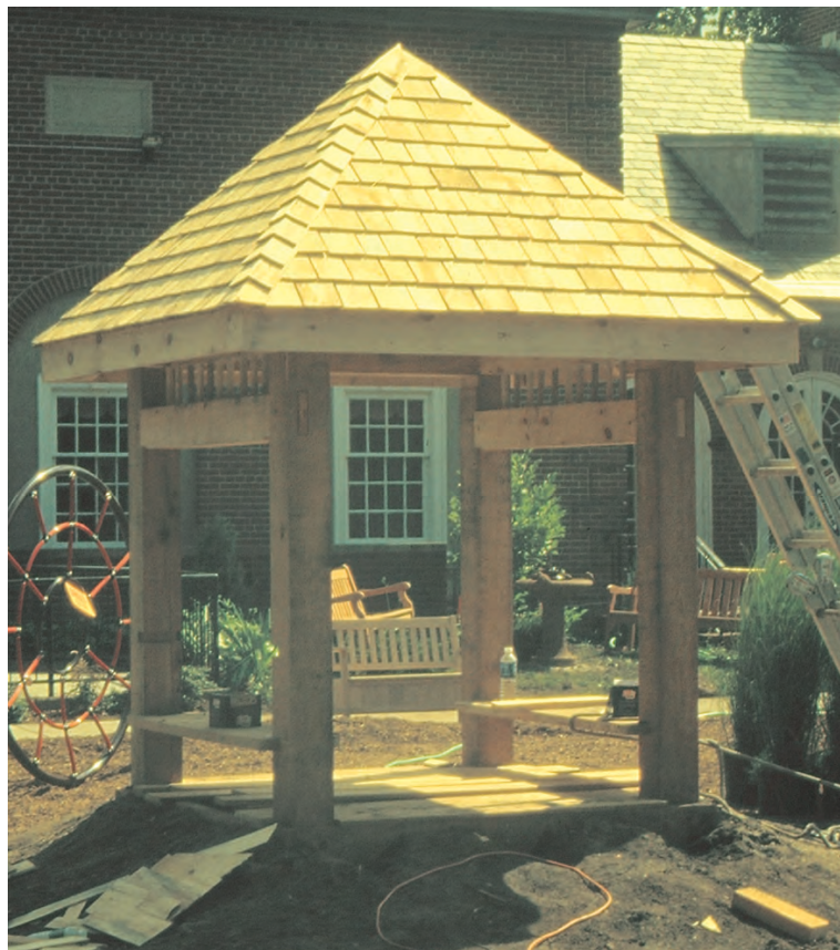
Fig. 8. Hip-roofed tower at Garden City, L.I. With no room for knee braces, the posts are fast in the ground and X-braced below grade.
