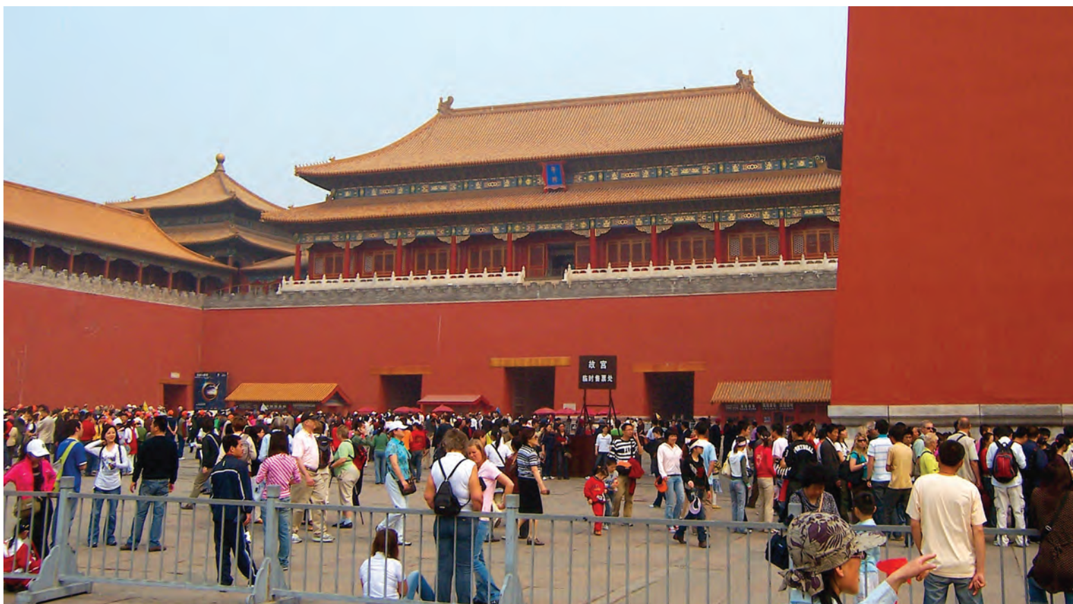
Fig. 3. Wumen (Meridian Gate), centered in south leg of city wall and formal entry to Forbidden City. In formal Chinese architecture, south is most auspicious cardinal point. Seven connected timbered halls (three visible) stand atop masonry and rammed-earth platform.
