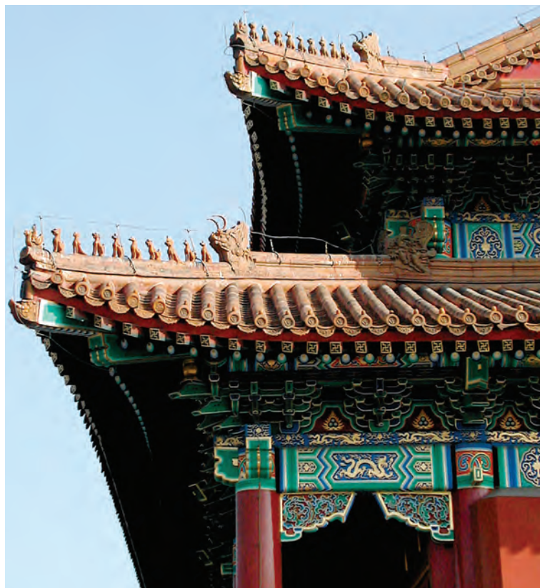
Fig. 14. Duanmen (Upright Gate). Double eaves show clearly upward slope when approaching hip. Round common and square flying rafters step progressively outward as well, creating curve in both elevation and plan. Flying rafters change from square to increasingly rhomboid as they approach hip.
