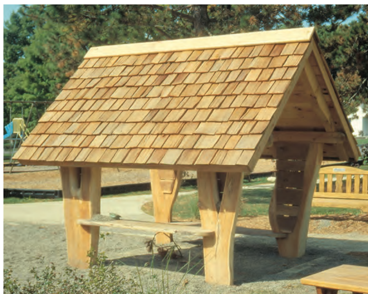
Fig. 6. Earthfast, forked locust posts blocked against head entrapment in playhouse, Ithaca, N.Y. Note integrated benches.
