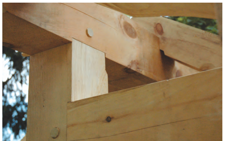
Fig. 4. Pegs are trimmed flush or proud enough to be easily spotted by kids but short enough to avoid creating a protrusion hazard.
