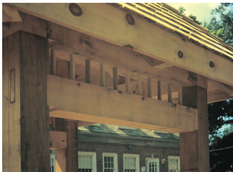
Fig. 5. Head entrapment in 5½-in. space between beams avoided by filling with 1-in. dowels, now a decorative feature.
