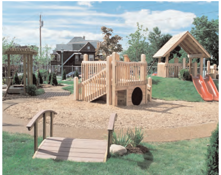
Fig. 2. Complex of pole- and timber-framed play structures built largely by volunteers for a childcare center in Watertown, N.Y. Wood fiber groundcover protects children from fall injuries.
