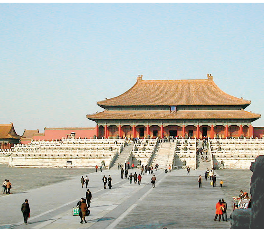
Fig. 7. Taihedian (Supreme Harmony Hall ) sits on a three-tiered carved marble platform with the typical three stairways. Thought to be the largest timber-framed structure in China, its double eaves and full hips express the formality expected of the emperor's main audience hall.
