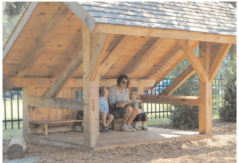
Fig. 3. At a Long Island daycare center, low tie beams with large 30-degree chamfers leave only 2 in. of flat surface, to avoid being considered a play surface that would call for shock-absorbent surfacing inside and outside the playhouse. But structure is incorrectly sited, too close to existing fence.
