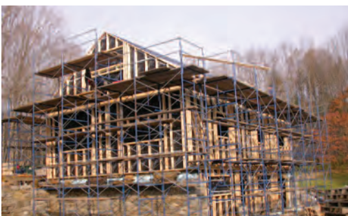
House frame built over barn frame.
