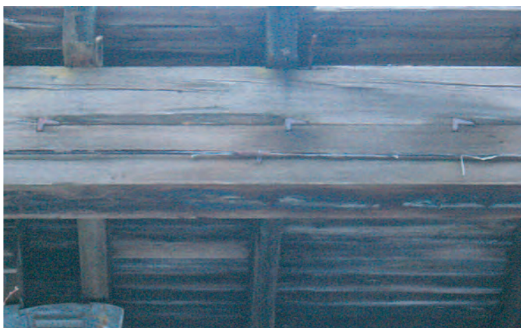
Ben Brungaber Fig. 12. Directional iron keys in built-up beam, West Lebanon, N.H.
