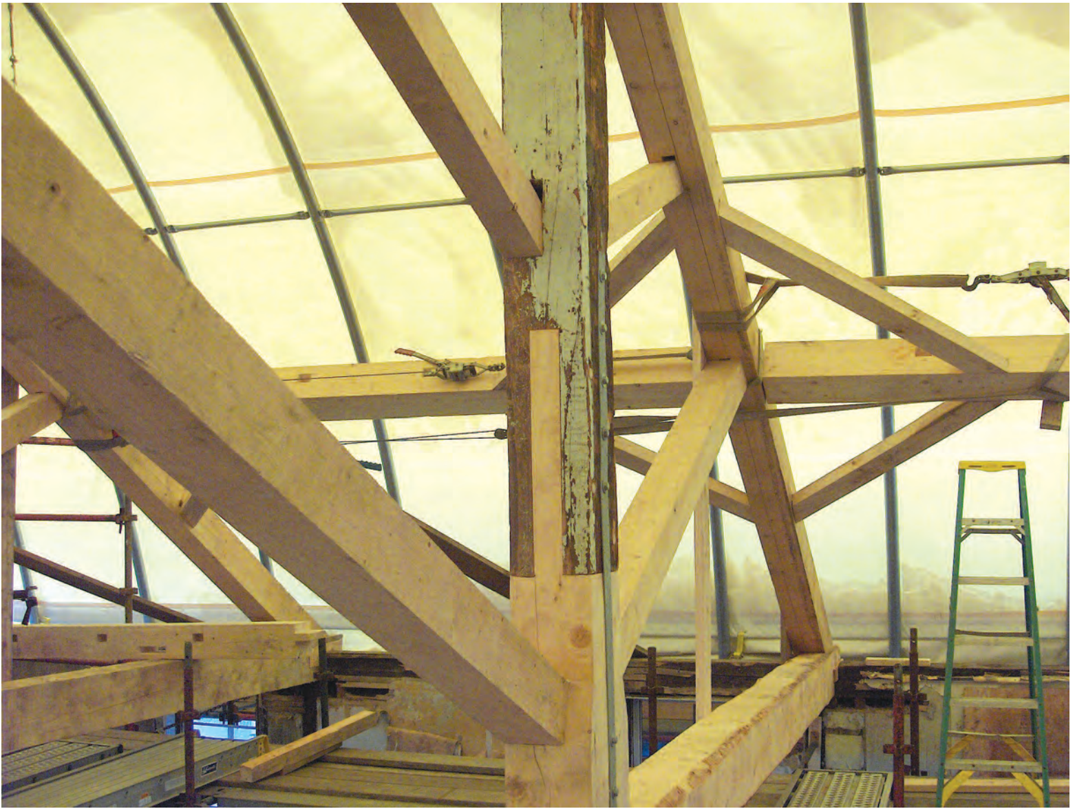
Fig. 8. Scarfed kingpost repair and extra-long stirrup strap to relieve tension at scarf. Trusses are double strutted and purlins are fully wind-braced. New timber is spruce. Translucent portable airplane hangar placed over building made work possible in almost any weather.
