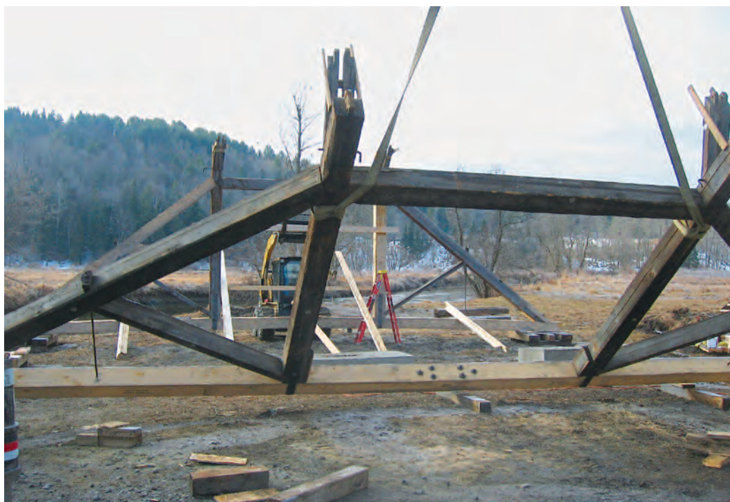
Fig. 6. Truss rising on blocking. Twinned braces prepositioned and strapped to top of queenposts, ready for tie beams. Portal bents will be added, then roof structure.
