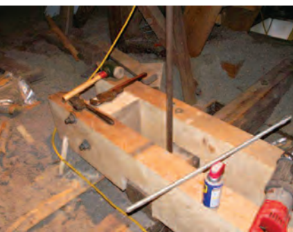
Figs. 3–4. Inner end of paired 5x12s, carried on lengthwise 8x8. At right, Chris Patton fits housed thrust block against truss rafter.
