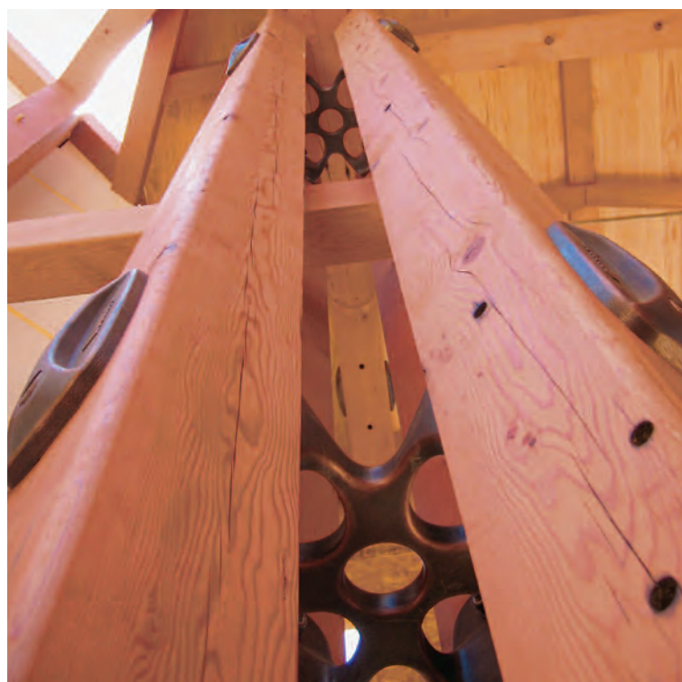
Fig. 14. At Wawona, California, cluster columns use housed decorative cast keys bolted through timbers to produce composite action.
