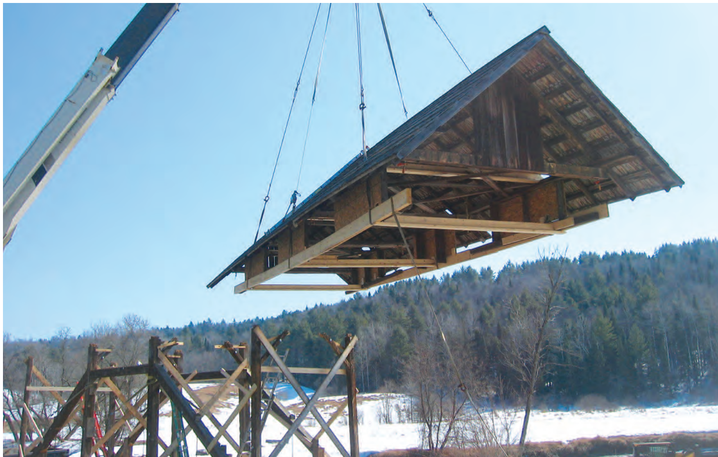
Fig. 2. Removing roof frame after bracing and reinforcement in place.
