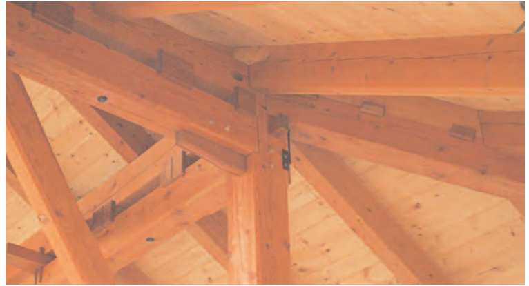
Fig. 18. Keyed hip and purlins meet at top of post at Massachusetts' Tewksbury Country Club. Purlin clamping bolts are spring loaded.
