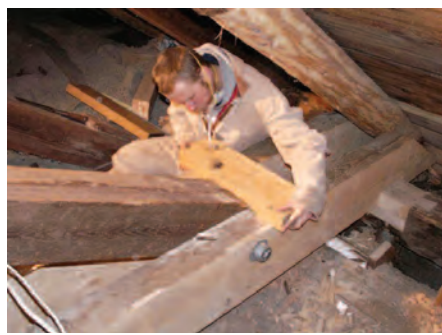
Figs. 3–4. Inner end of paired 5x12s, carried on lengthwise 8x8. At right, Chris Patton fits housed thrust block against truss rafter.
