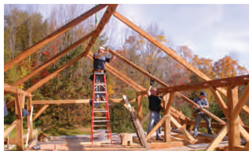
Tenoned rafters brought up one by one.
