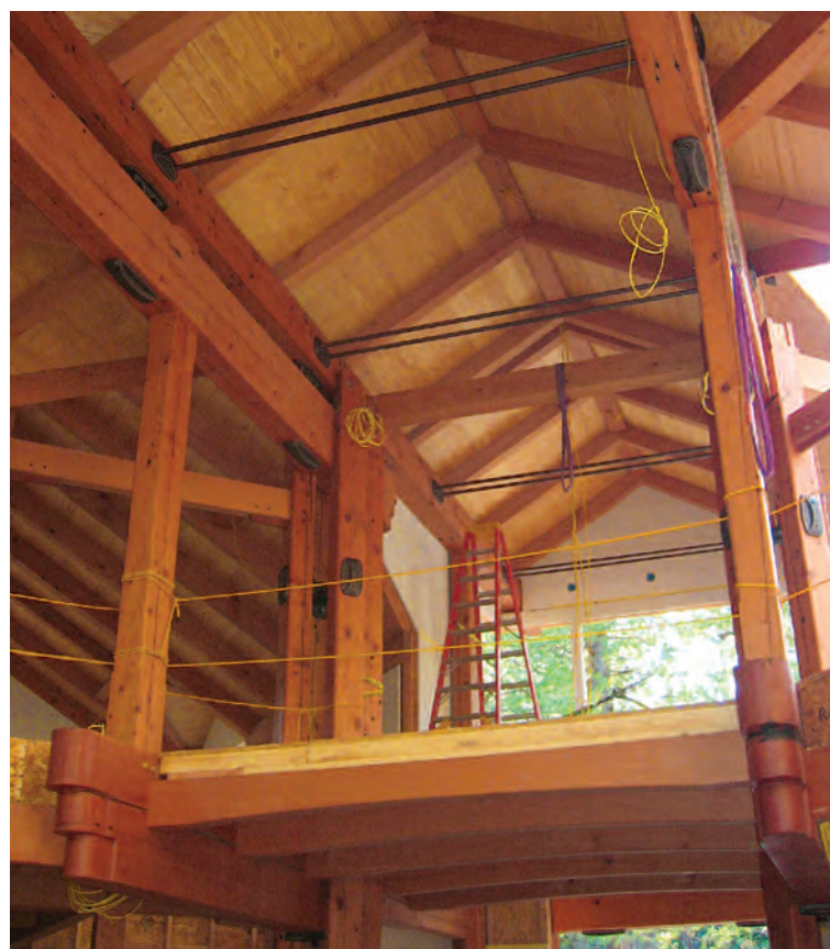
Randall Walter AIA Fig. 15. Elaborate washers seen on keyed beams and posts are cast in same style as keys. Decorative ends are cut on solid recycled beams.
