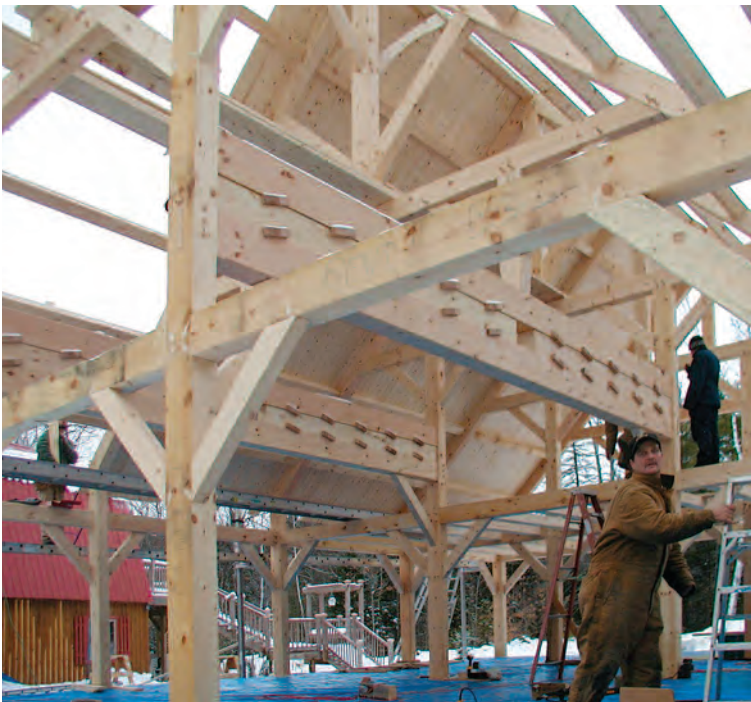
Fig. 17. In New Hampshire, triple-laminae white pine beams with sloping, folding-wedge keys. Gaps in central lamina fall at area of no stress and will be occupied by a tie beam joining the keyed beams.
