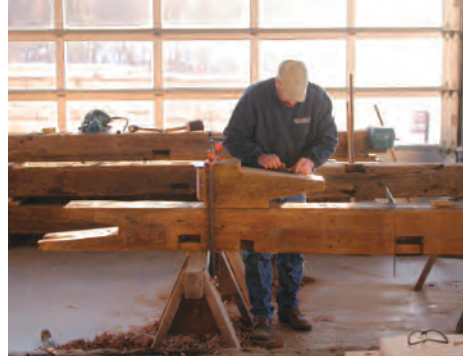
Post repairs in shop and installed in restored frame. Gerard Laflamme at left, Mike Fountain above.
