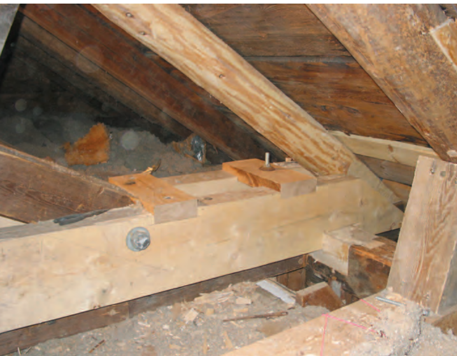
Fig. 5. Heavy bolt clamps paired 5x12s to truss rafter, shares thrust with housed oak block. New shaved end for round common rafter, dovetailed patch for plate just visible under nearer 5x12.
