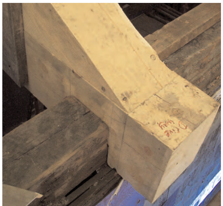
Fig. 9. Intermediate lower chords lap the continuous plate.
