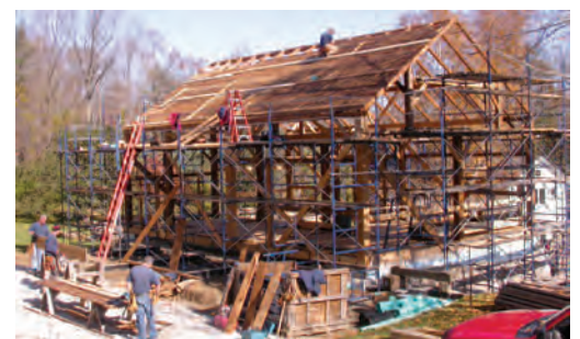
Staged up for roof boarding.
