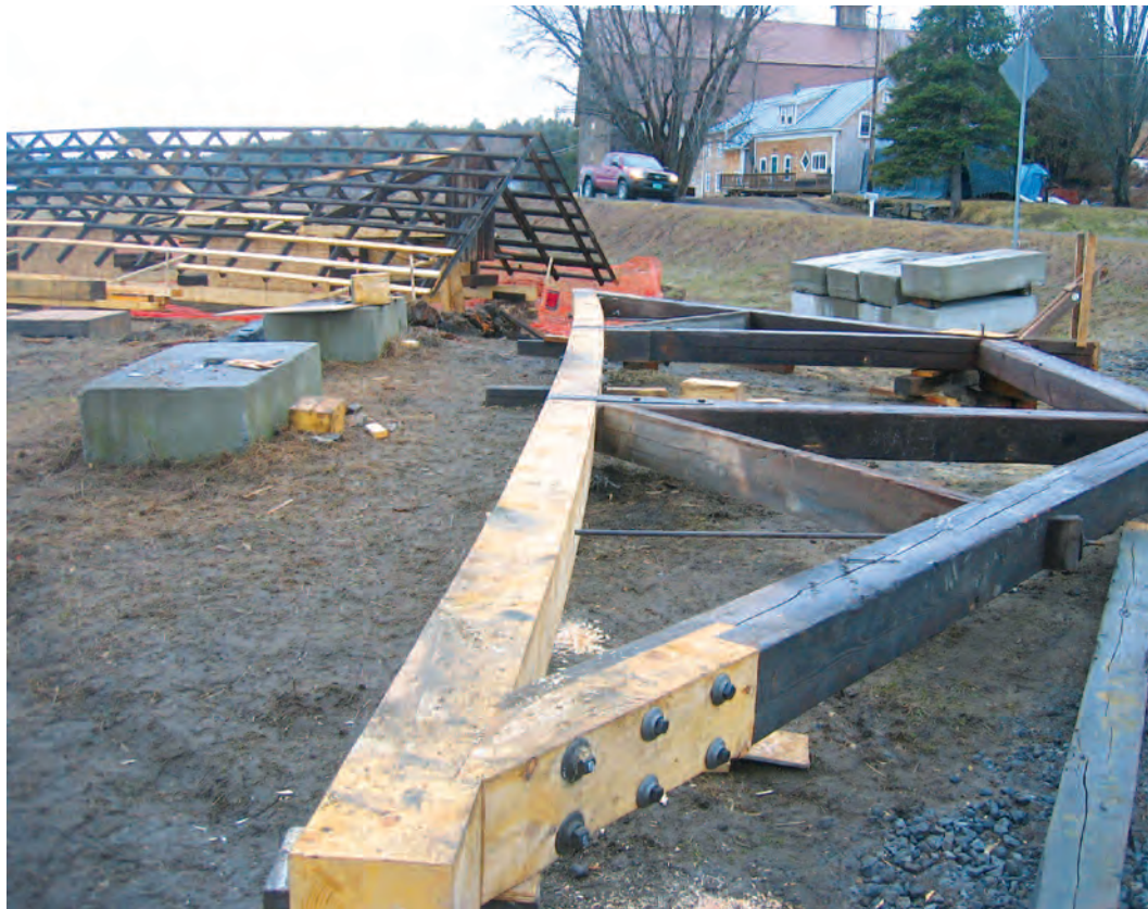
Fig. 5. New cambered chord and repaired main brace in reassembled queenpost truss.
