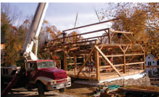
Purlin posts, purlins and roof ridge added.
