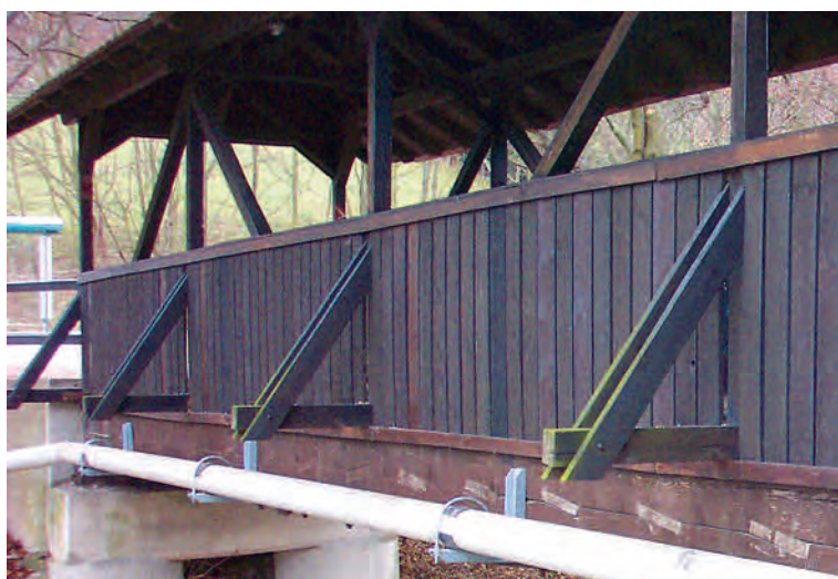
Fig. 8. Bridge in Austria relies on sloped-key-laminated girders for load bearing. Diagonal members in “truss” brace roof structure only.
