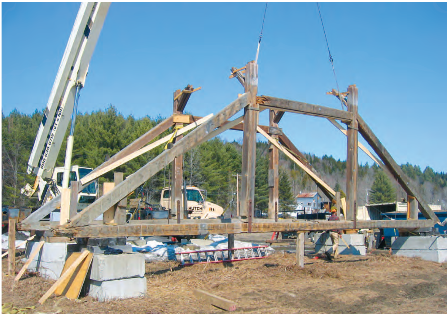
Fig. 4. Trusses exposed. Note heavy stirrup straps at bottom of queenposts and short, twinned braces at top. Struts between main braces and queenposts have been removed. Original camber in scarfed bottom chord has disappeared. All timbers tagged with disks.
