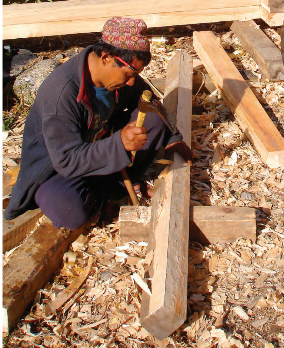
Fig 9. Orgun Grung hand-adzes a roughsawn timber to size, hewing to struck line. Timber will later be bench planed.
