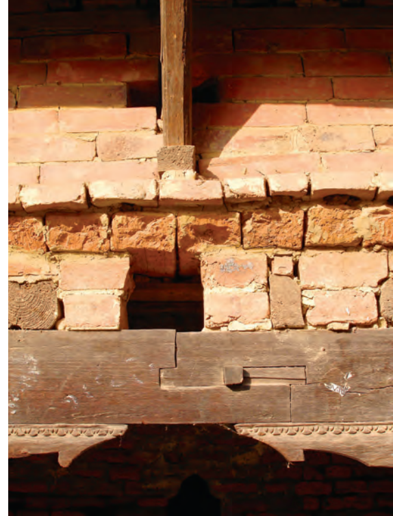
Fig. 6. Cholu scarf joint in pati beam, Patan.
