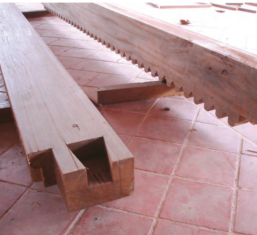
Figs. 18–19. New Shiva temple, Pokhara. Dovetailed timbers are horizontal exterior beams to be located above brick façade and at feet of the struts, oriented with marriage marks on top and dentil carvings facing out, forming a horizontal band (cf. Fig. 15). The temple will have a two-stage roof with corresponding proportions of perimeter beams and struts.
