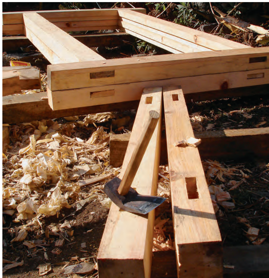
Fig. 10. Through mortise and tenon door and window frames.
