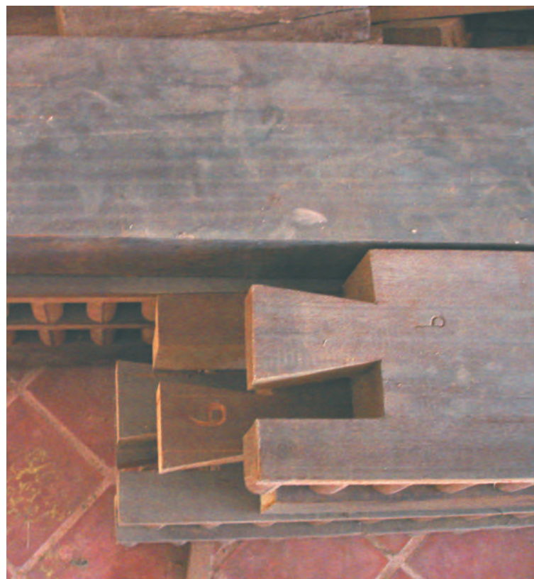
Figs. 18–19. New Shiva temple, Pokhara. Dovetailed timbers are horizontal exterior beams to be located above brick façade and at feet of the struts, oriented with marriage marks on top and dentil carvings facing out, forming a horizontal band (cf. Fig. 15). The temple will have a two-stage roof with corresponding proportions of perimeter beams and struts.
