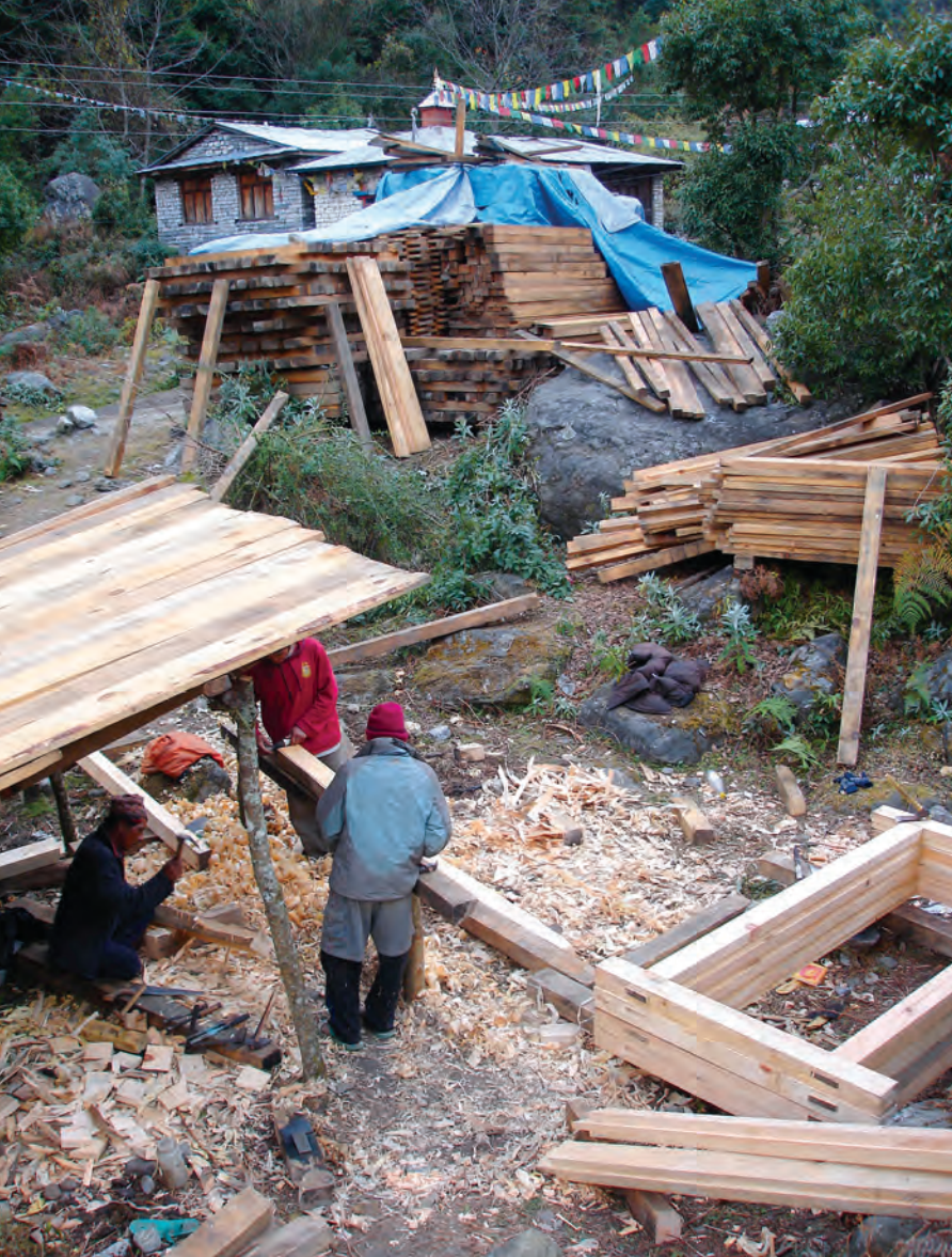
Fig. 11. Carpenters' yard at Danakyu, elevation 2300m. Lining one roughsawn timber on bench while another is sized with adze. It will be finished with a long plane.
