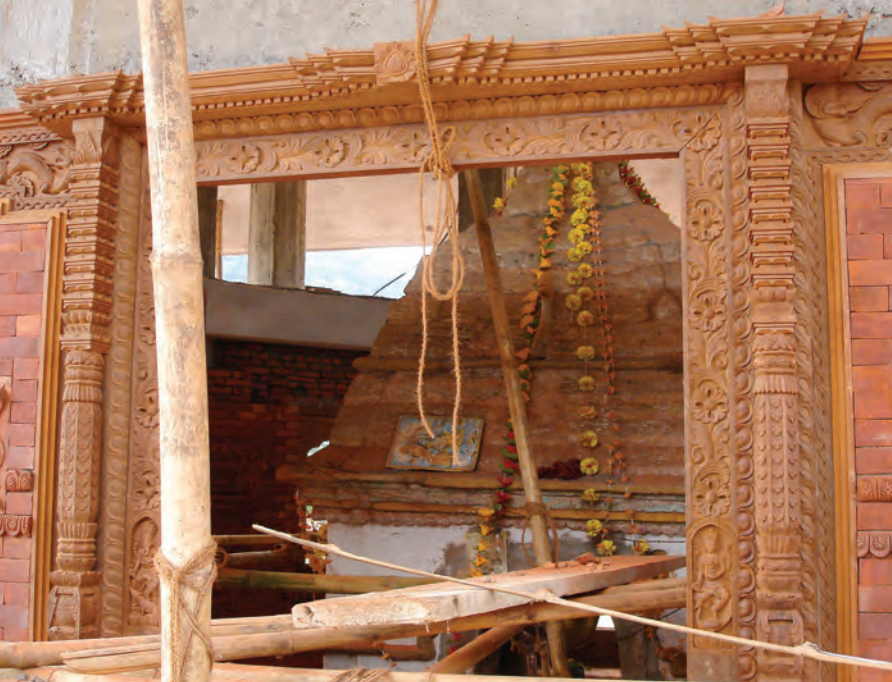
Fig. 16. Carved timber elements, entryway of new temple in Pokhara. Body of temple is concrete and brick. Note bamboo scaffolding.
