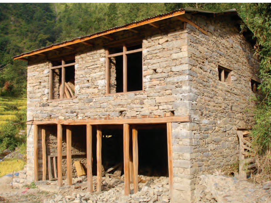
Fig. 1. New house near Balphi. Framing below for shop-front doors.
