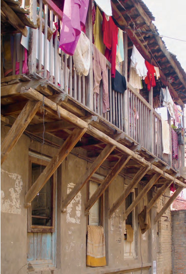
Fig. 8. Diagonal struts support both balconies and large roof eaves. Note double scarf joint at middle of jetty sill.
