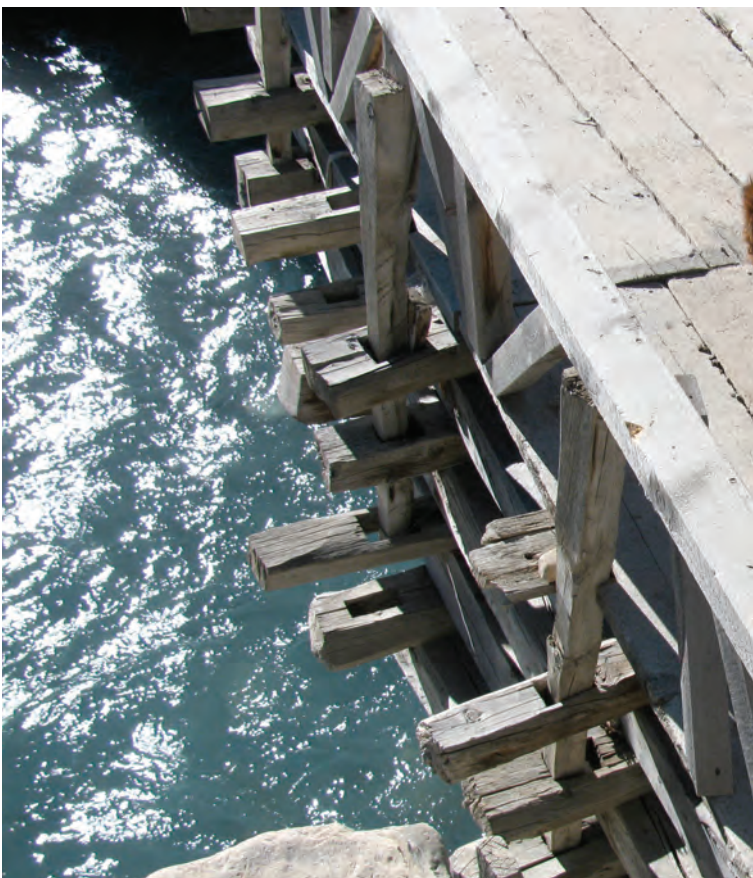
Fig. 14. Vertical needles thread through successive crib ends. Independent railing appears not to contribute to bridge stiffness.
