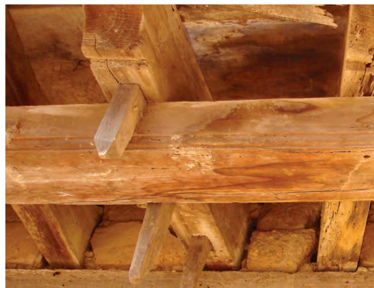
Fig. 7. Stout square pegs ( chuku ) often locate one beam on another.
