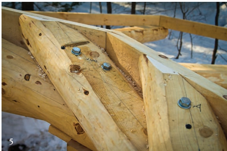
3 First two rafters supported by future temporary winter post.
