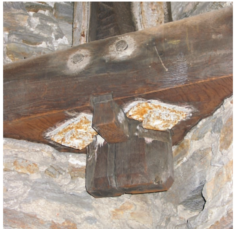
14 Christ Church, Philadelphia, 1760, lower terminus of composite steeple stage tie down.
