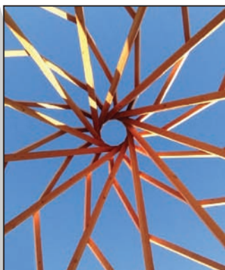
Reciprocal roof framing at the St. James Episcopal Church in Cannonball, ND by Empire Timberworks.
