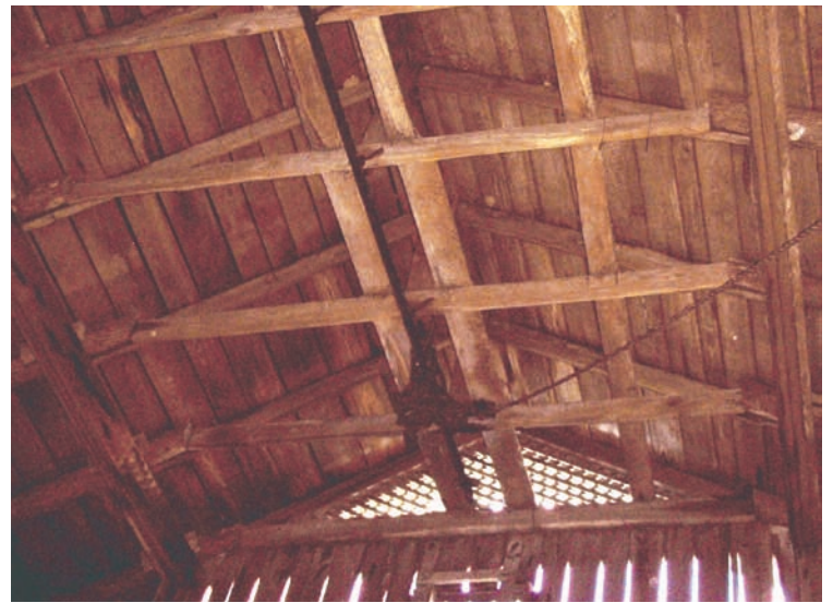
7 Hay car, extended rafters and scalloped siding (Saylor barn).
