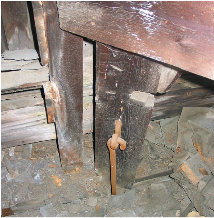
6 Above, Bethany Church, wrought-iron hold-down rod attached to spire rafter foot and bell deck timber a stage below.
