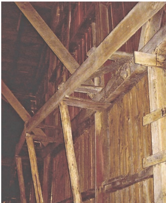
9 Gable end of widened barn stiffened against wind by shallow horizontal truss, seen in most split barns at both ends at or near tie beam level.
