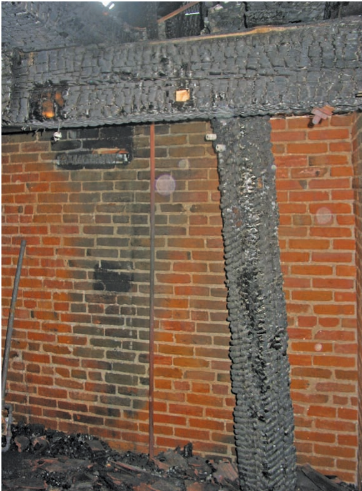
11, 12 Above, charred sleeper still in place at top of College Street tower, spire rafters gone. Tie-down rod drops 8 ft. to bell deck framing below. At right above, cut fragment of sleeper and plate, mortise and housing on top surface skewed for octagonal-spire rafter foot.
