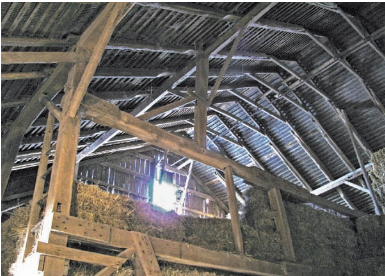
6 Rafters extended after splitting, posted purlin under long run.
