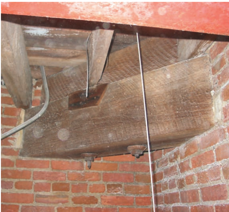
13 College Street descending timbers, not pendant as at Bethany, but firmly bolted at their feet to short stout members embedded in corners well down in masonry tower.
