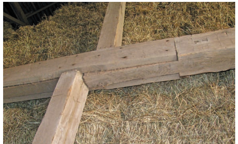
8 Oak tie beam splice, roughly fashioned after barn splitting.
