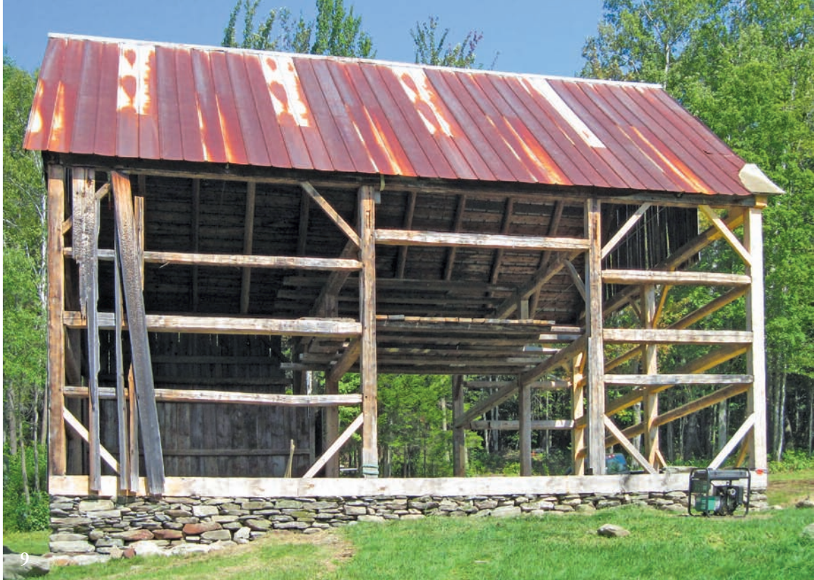
5 At left, Slayton barn roof framing, first quarter 19th century, Calais, Vermont. Long brace let in to tops of rafters similarly to Fitch barn in same town.
