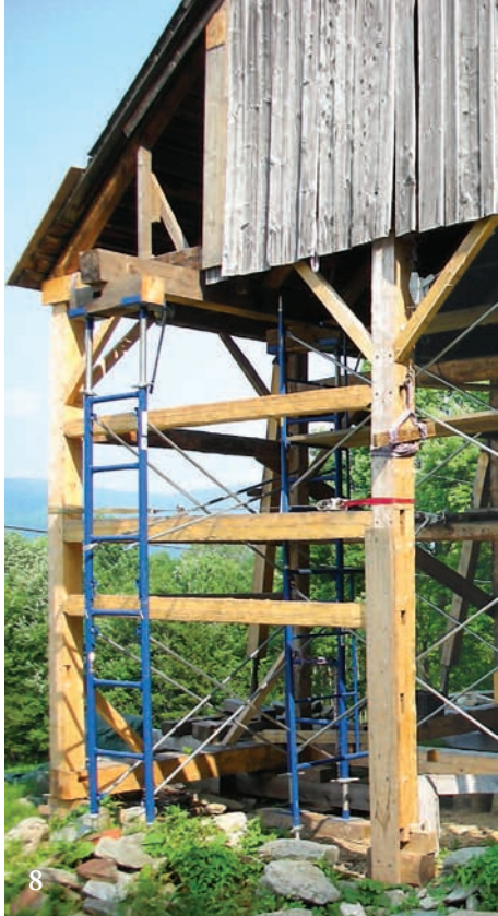
5 At left, Slayton barn roof framing, first quarter 19th century, Calais, Vermont. Long brace let in to tops of rafters similarly to Fitch barn in same town.
