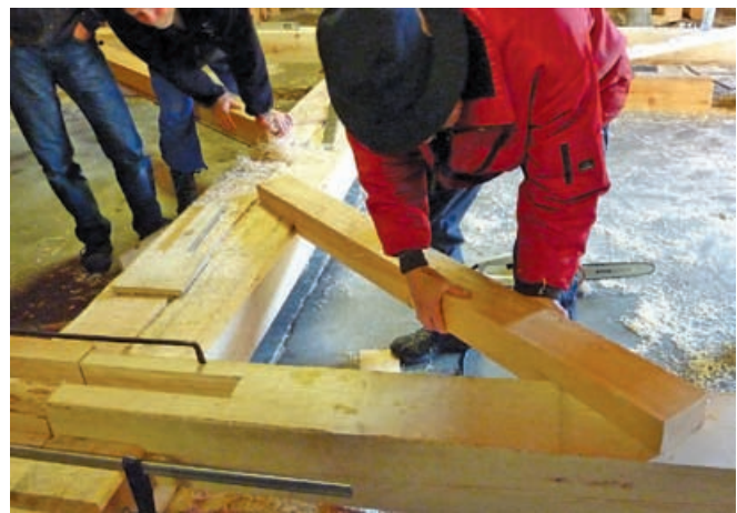
14 Brace located, Kåre Herfindal marks for shoulder. 15 Shoulders cut, tenons to scribe on post and plate.
