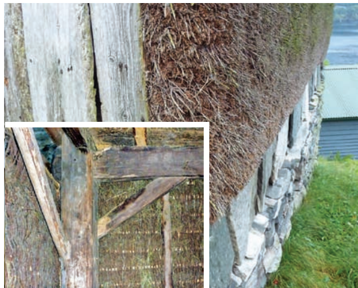
21 Juniper woven on poles (inset) clads grindbygg near Bergen.
