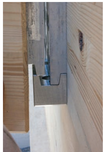
3 Detail of mating connectors and lower clamp jaw.
