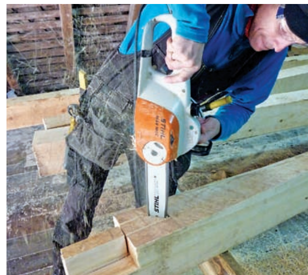
20 Chainsaw in skilled hands cuts or roughs out joints.
