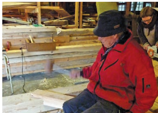
16 Tenon outline scribed, depth marked with template. 17 Lap housings cut, Kåre hammers home brace.
