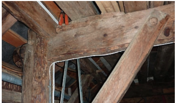
13 Piece pegged to top of tie beam serves to keep plate tight to post. Wedge has gone missing with no sign of subsequent plate movement.
