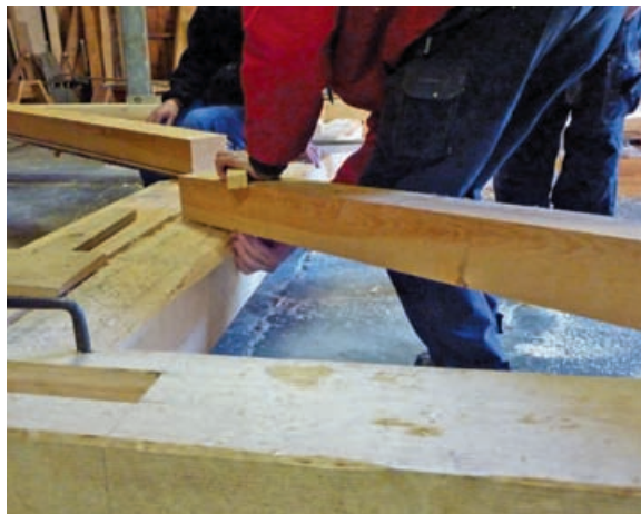
14 Brace located, Kåre Herfindal marks for shoulder. 15 Shoulders cut, tenons to scribe on post and plate.
