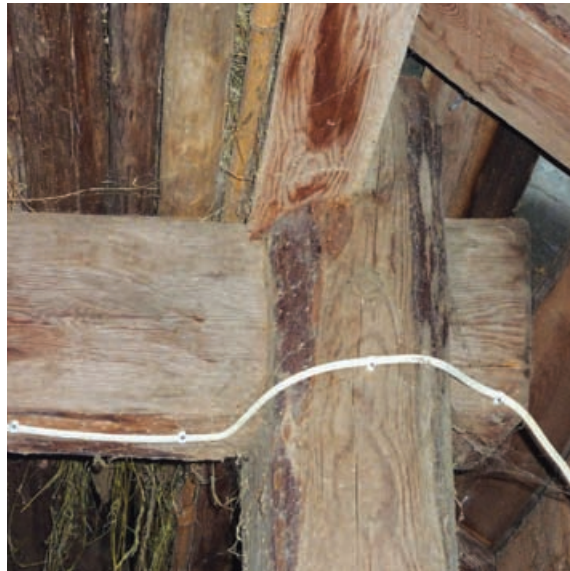
11 Large peg set in tie beam just inside plate helps keep plate from rolling under rafter action. Note step-lap rafter joint.
