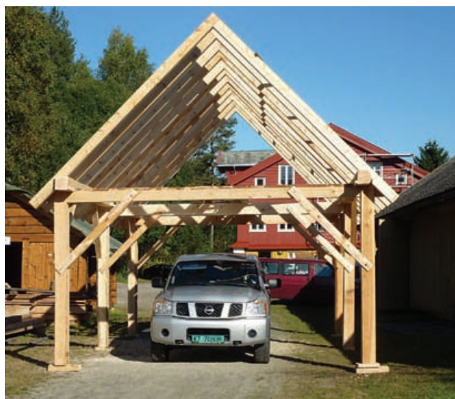
4 Class-built grindbygg frame, in service as carport, Voss.
