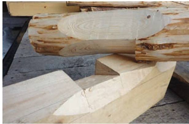
18 Inverted-V in plate provides easily cut rafter seat.
