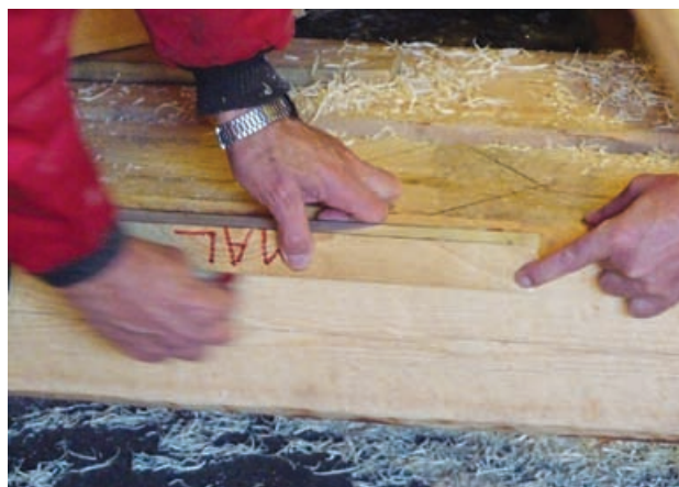
16 Tenon outline scribed, depth marked with template. 17 Lap housings cut, Kåre hammers home brace.
