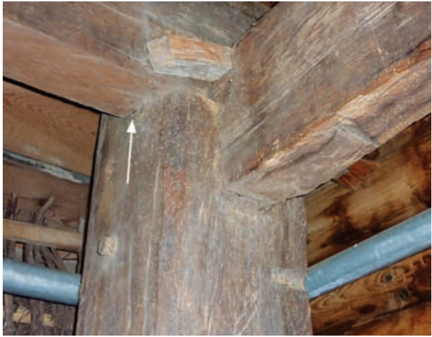
9 Plate (at back of photo) notched to tie and post (arrow). Notch for post fairly shallow.
