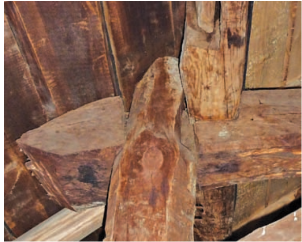
9 Plate (at back of photo) notched to tie and post (arrow). Notch for post fairly shallow.
