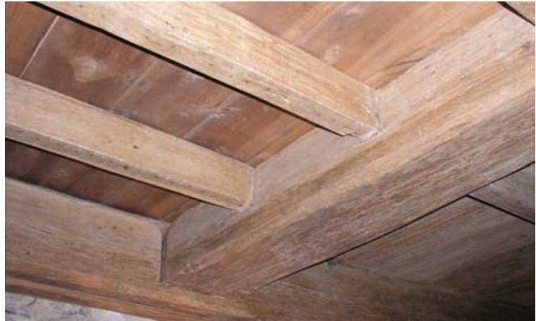
1 Tenoned oak floor joists and carrying timber, Guilford Ct., 1646.
