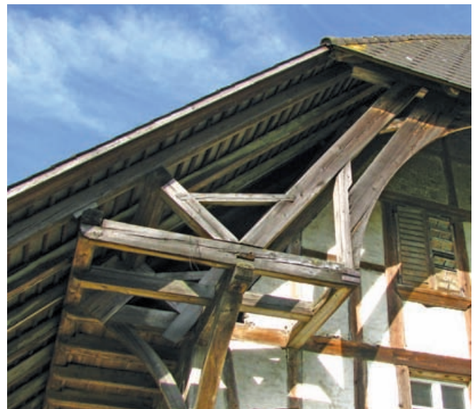
8 Representative overhang framing with outer rafter loads balanced over indicated support points.
