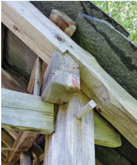
11 Large peg set in tie beam just inside plate helps keep plate from rolling under rafter action. Note step-lap rafter joint.
