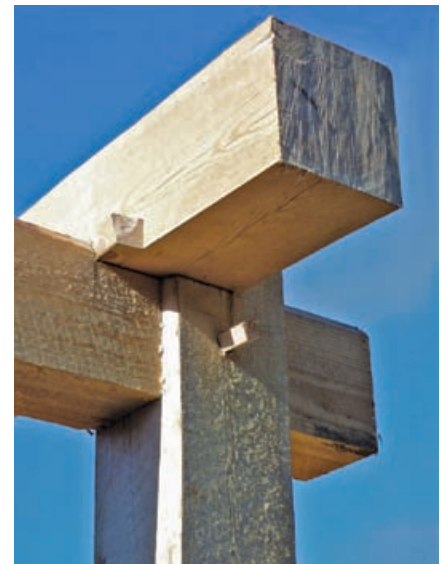
7 At left, exploded view and anatomy of necked tying joint, here with folding wedges to restrain lower part of plate against rafter action that ultimately locks joint.
