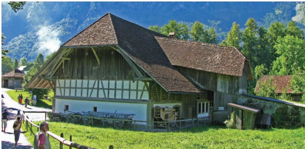
3 Agricultural portion of same 1797 Bernese farmhouse. Note partly covered access ramp to hay mow (on right), broad and complex overhang framing, open slats for crop ventilation along eaves walls, utilitarian wall boarding, masonry construction of lower level.
