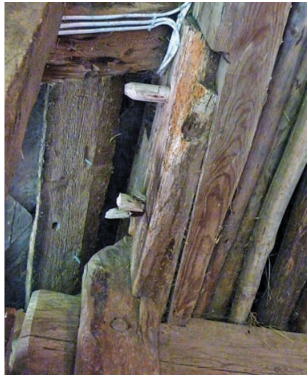
19 Antique stop-splayed and pegged scarf.
