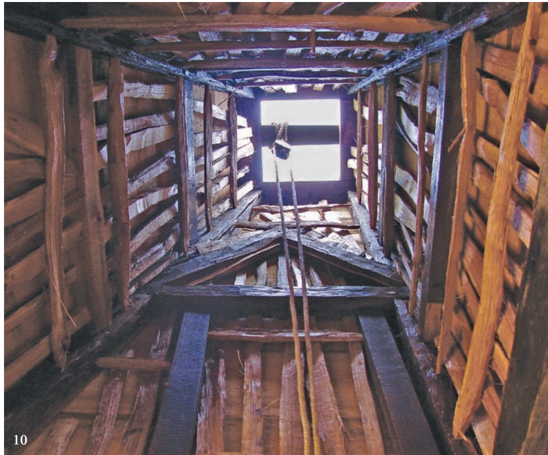
10 Chimney framing integrated with end wall of house. Note collar beam, studs, end rafters. Pulley wheel and rope allowed mason to haul daub bucket to top to start job, then to any point below.
