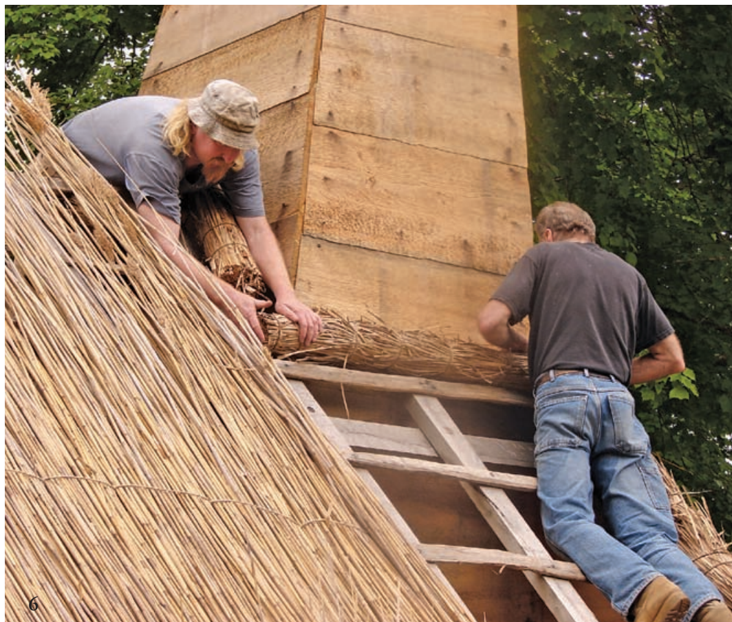
6 Thatchers Michael French of Plimoth Plantation and Lorin Johnson, a friend of the Knight House team, place bundled rolls at chimney base to hold next layer. Bundled rolls surround chimney and roof perimeter.
