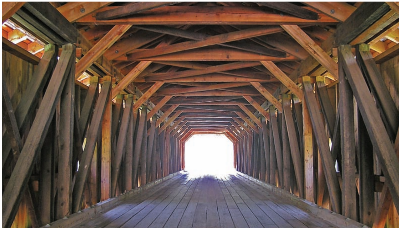
Hamden Bridge, Delaware County, New York, 128-ft.-span Long truss built over Delaware River in 1859 and propped midspan by pier in 1940s. During rehabilitation in 2000, pier was removed and bottom chords replaced by glulam because of theoretical weakness of chord splices, even if in good condition, in original design.
