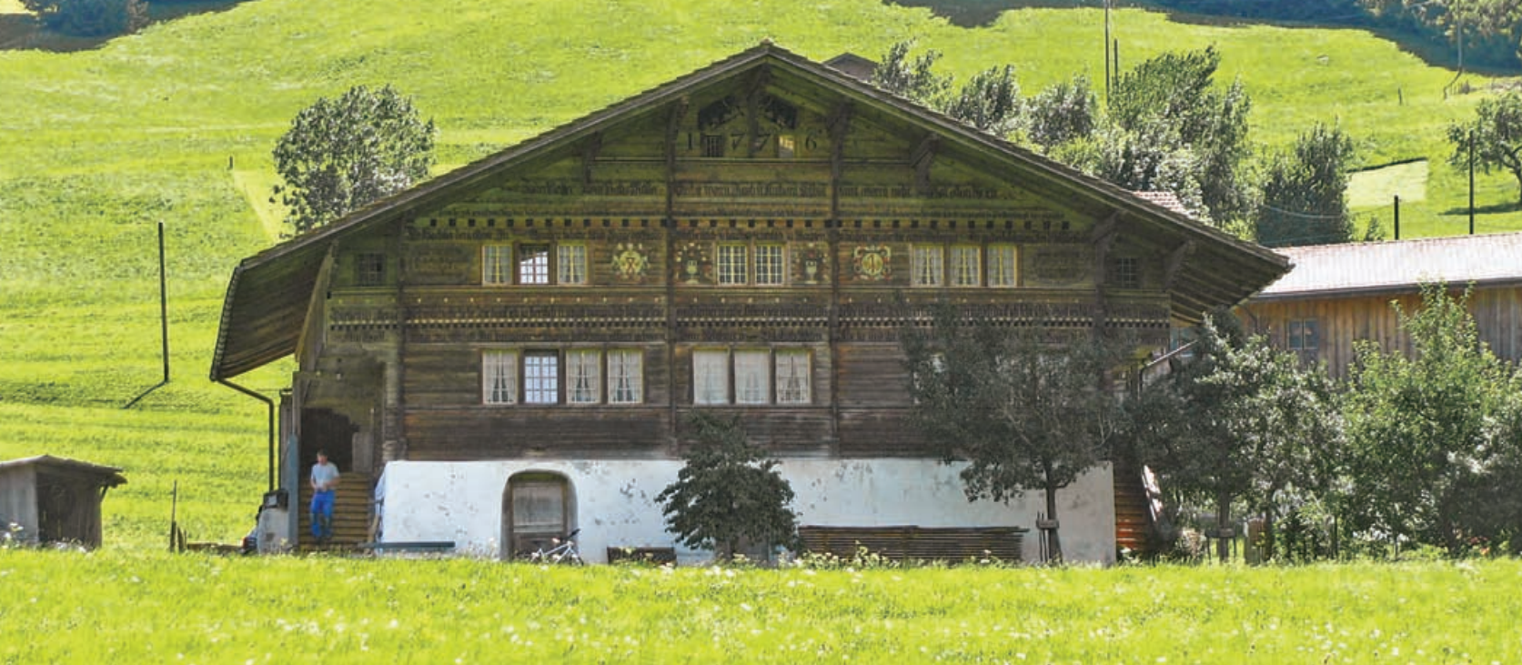
1 Typical Oberland house, built 1776, with plastered masonry walkout cellar, squared log construction above, usually of fir or spruce.
