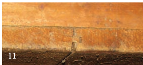
9, 10, 11, 12 Single beam, the Unterzug , spans width of room, supports plank floor. Course of projecting timbers grooved on inner faces, the Bund , holds planks' edges and ends around perimeter of room. Planks meet in tongue-and-groove or loose-tongued ( Heidendecke ) joints. Central plank in floor, wedge-shaped, is driven from outside of building to tighten floor and left proud to continue tightening as necessary.
