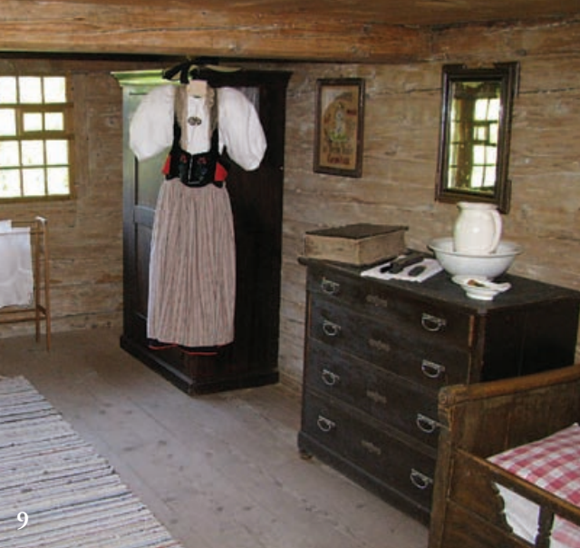
9, 10, 11, 12 Single beam, the Unterzug , spans width of room, supports plank floor. Course of projecting timbers grooved on inner faces, the Bund , holds planks' edges and ends around perimeter of room. Planks meet in tongue-and-groove or loose-tongued ( Heidendecke ) joints. Central plank in floor, wedge-shaped, is driven from outside of building to tighten floor and left proud to continue tightening as necessary.
