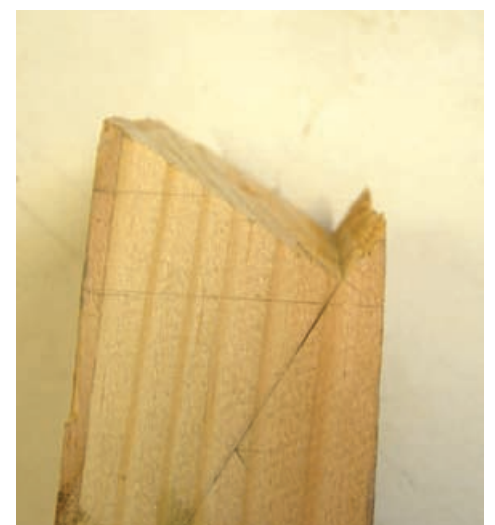
17 At left, the hip laid out, ready to cut.
