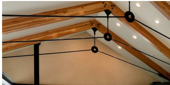
Photo 1 - King-rod truss roof framing
